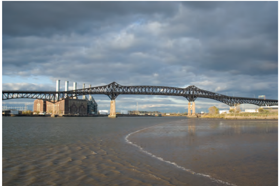
Plan 2035 calls for repair and maintenance of the region's many bridges. Pulaski Skyway, Essex and Hudson counties.
