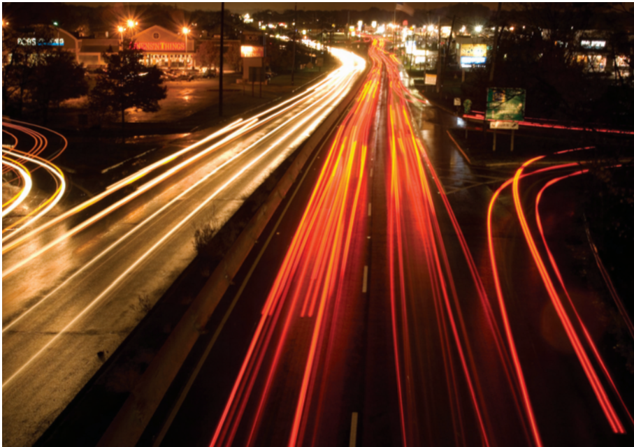
North Jersey's heavily traveled, aging transportation system poses a difficult funding challenge to the region. Route 22, Springfield, Union County.
