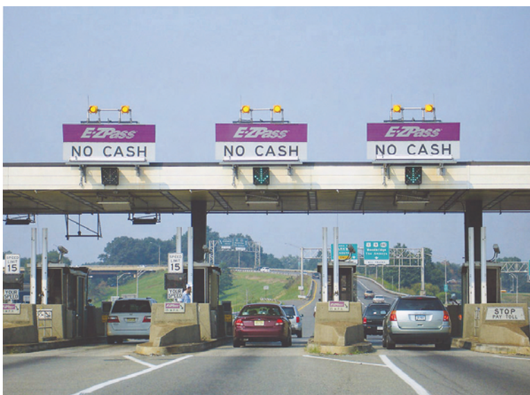
Toll plaza on New Jersey Turnpike, Middlesex County.
