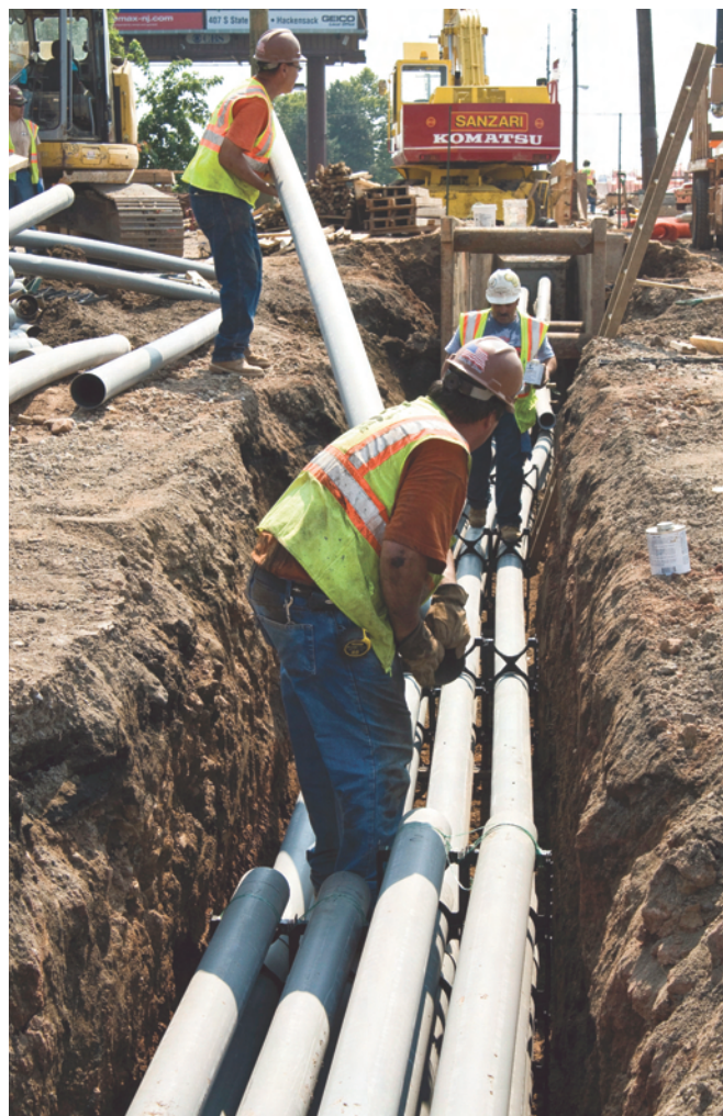
The American Recovery and Reinvestment Act funded dozens of projects in the region. Lodi, Bergen County.
