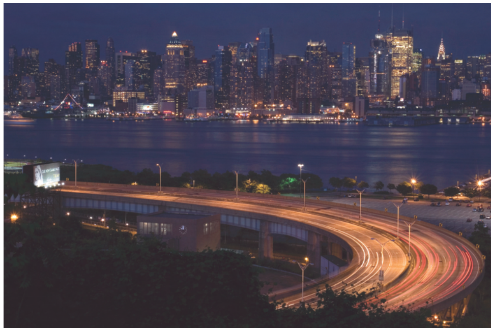
Toll facilities are just one way the region can generate revenue for transportation investments. Helix approach to Lincoln Tunnel, Weehawken, Hudson County.
