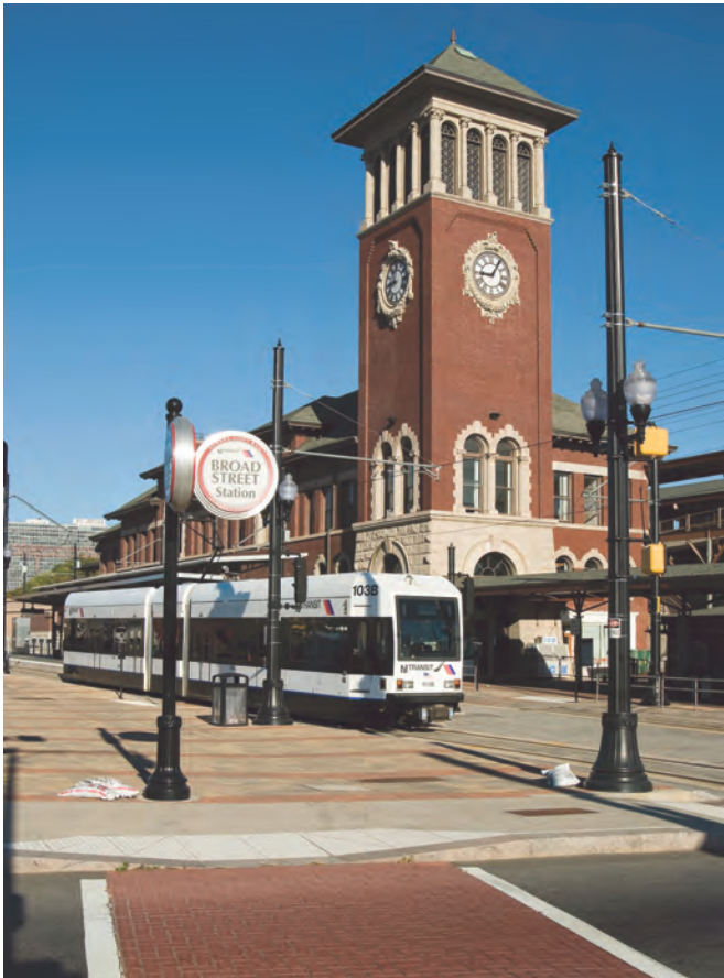
Light rail provides an alternative mode of transportation in urban areas. Broad Street Station, Newark.
