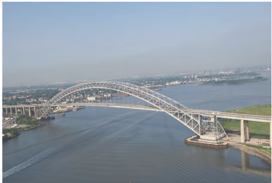
The region must address the limited clearance under the Bayonne Bridge to remain competitive in a changing global marketplace.
