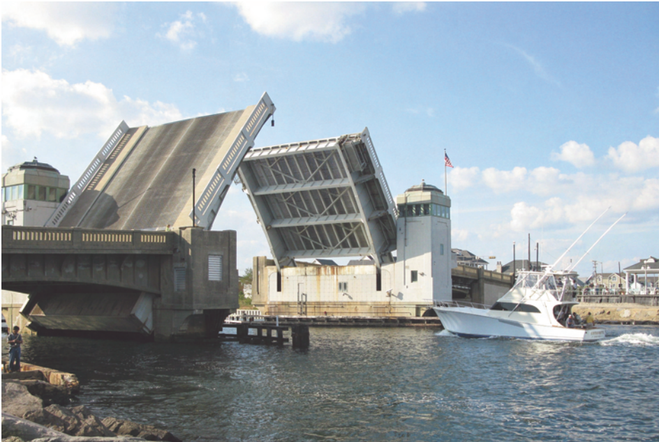
The NJTPA's extensive coastal areas have unique transportation and environmental needs. Shark River Inlet, Monmouth County.
