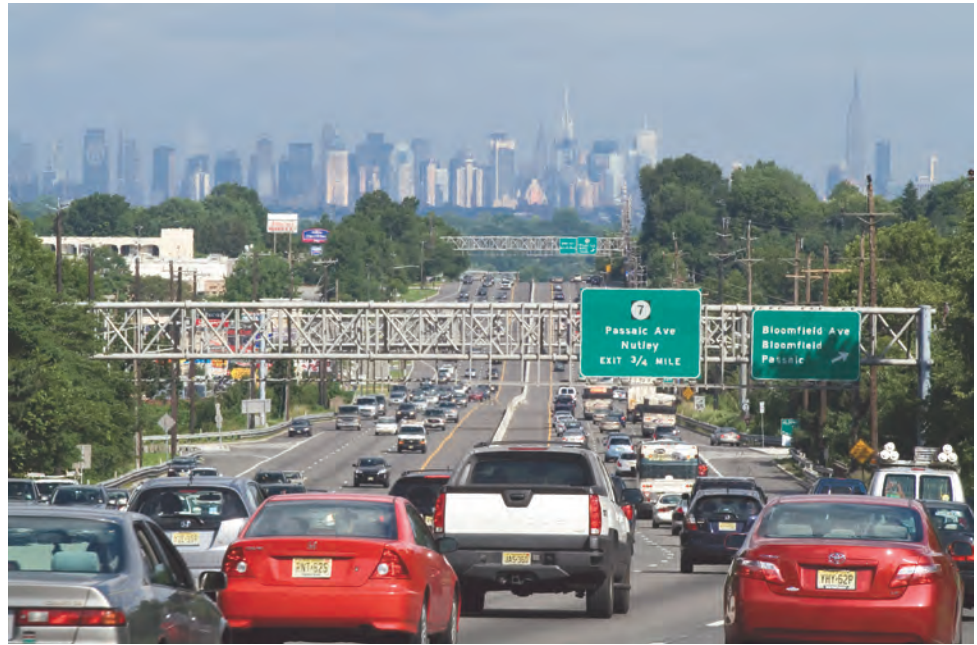
Plan 2035 seeks to address key congestion hotspots and to make the region's road system handle traffic more efficiently. Route 3, Passaic County.
