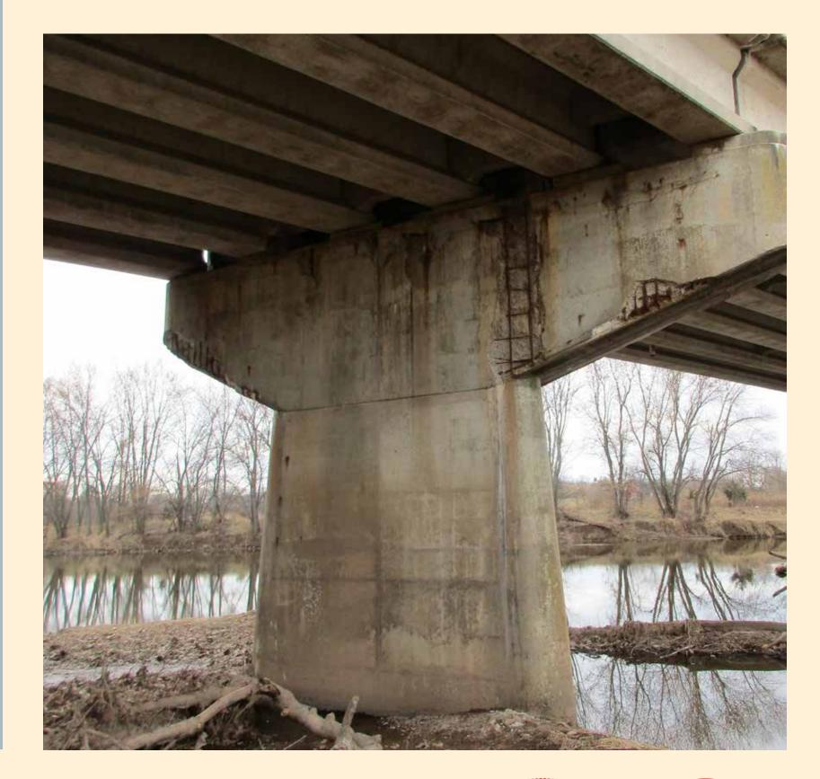
Built in 1979, the bridge is classified as structurally deficient and functionally obsolete. The concrete is deteriorating, resulting in rusting of the reinforcing steel substructure.
