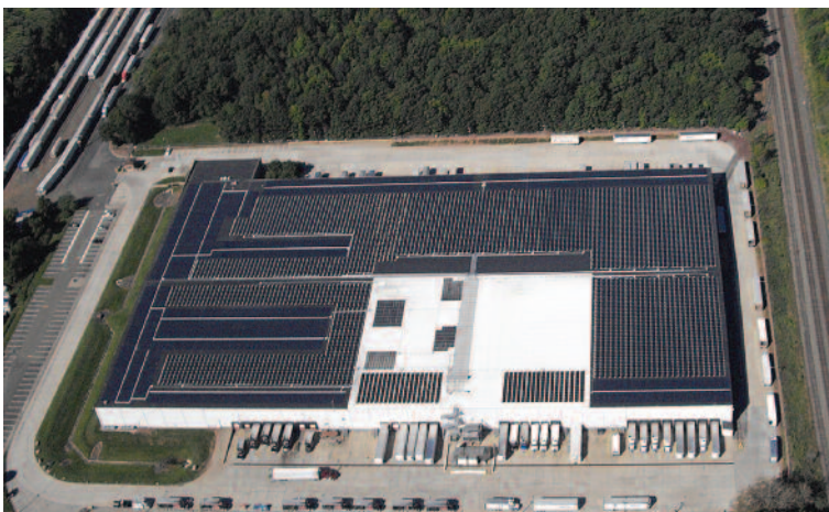
Rooftop and aerial views of one of Hall's Warehouse Corp.'s three facilities in South Plainfield, Middlesex County.
