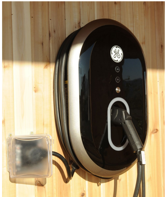
Photo by Thomas Kelsey, NREL 37699
