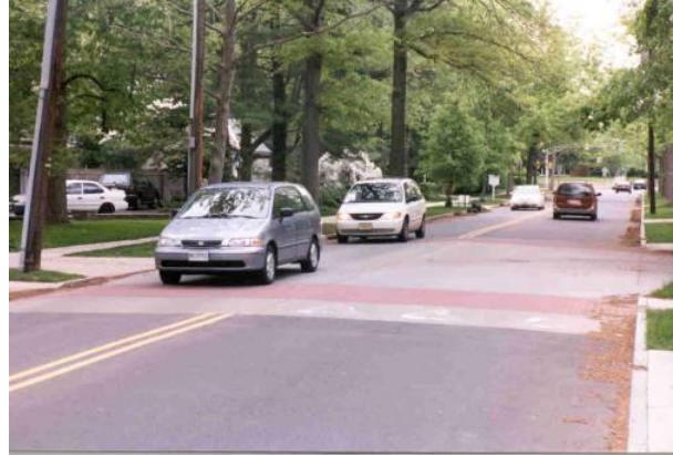
Figure 2: Example of a raised crosswalk in Princeton, N.J.
