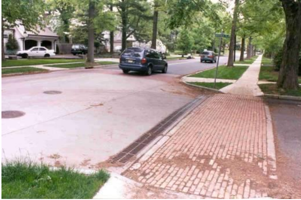
Figure 2: Example of a raised crosswalk in Princeton, N.J.
