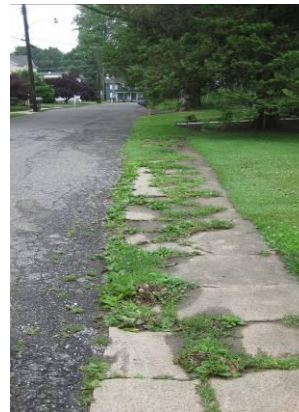
Center St. facing north
