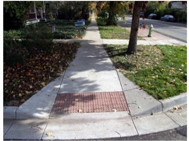
ADA Compliant Curb Ramps
