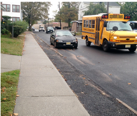
Curbing is greatly diminished or non-existent along River Drive.
