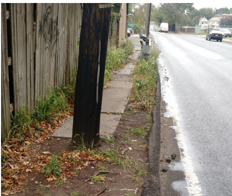
Sidewalk ends and utility pole interrupts pedestrian way.
