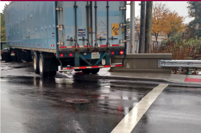
Figure 20: Truck Encroaching on Curb
