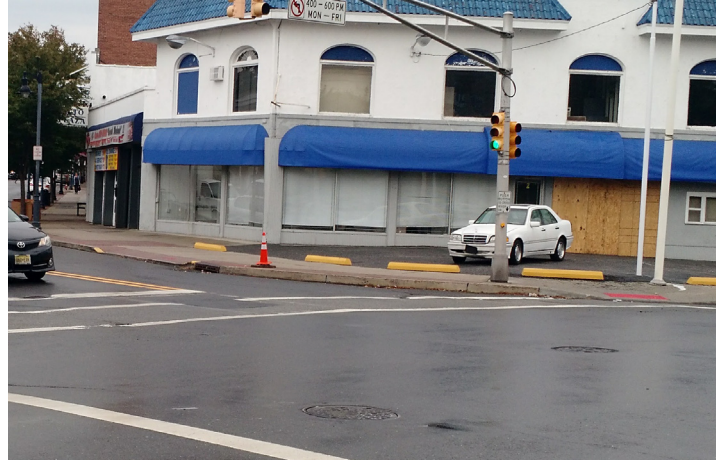
Figure 49: Parking Blocks Prevent Cars from Encroaching on Sidewalk
