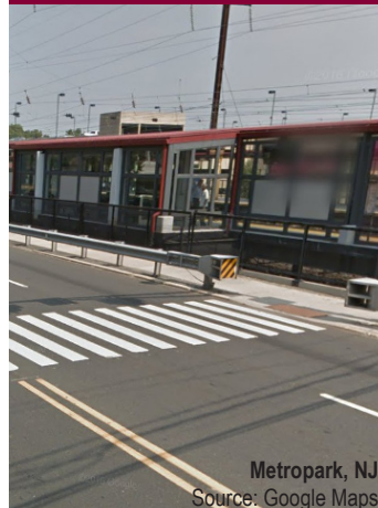
Figure 52: High Visibility Crosswalk
