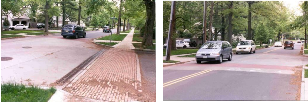
Figure 4: Example of a raised crosswalk in Princeton, N.J.
