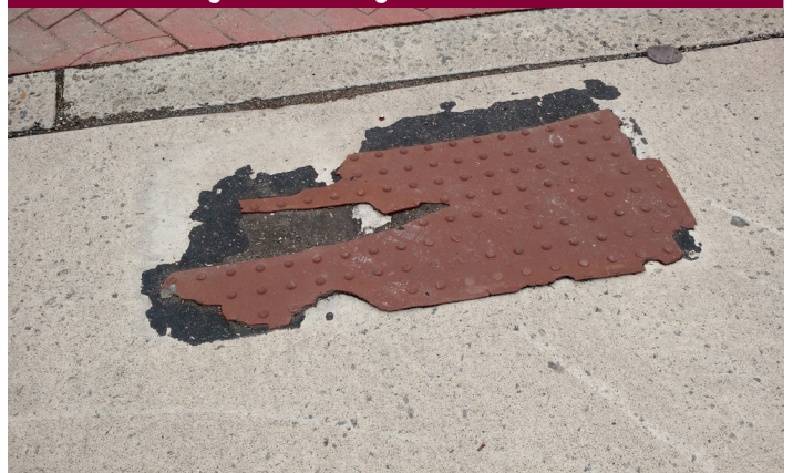
Figure 14: Damaged truncated dome
