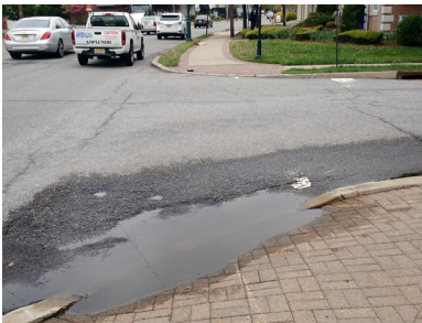
A lengthy depressed curb exposes pedestrians to vehicles backing up for a longer distance than a standard 24-foot driveway. Vehicles backing into the travel lane may also pose a safety concern for drivers.
