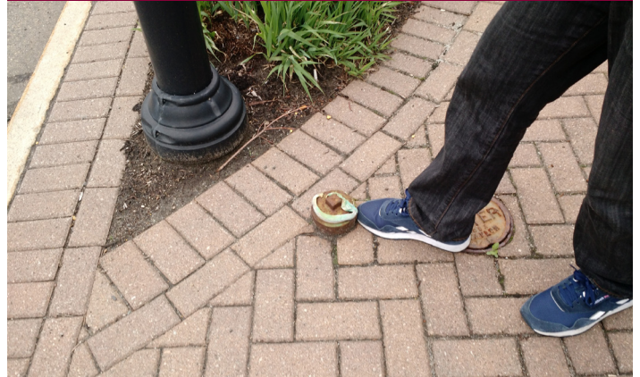
Figure 14: Damaged truncated dome
