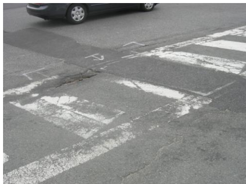
Repaint crosswalks and eliminate 'spot' hazards in pavement.
