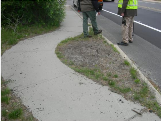
Eliminate curves in sidewalk that could cause difficulties for accessibility.
