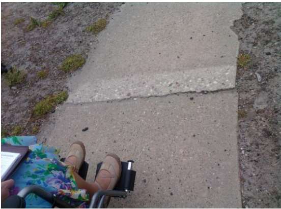
Eliminate uneven pavement hazards causing difficulties for accessibility.
