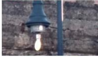
Exposed light bulb.
