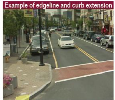
The group discussed the many different forms of curb extensions, from the low-cost, quick fix extensions with texturized paint and bollards to poured concrete extensions such as those immediately above.
