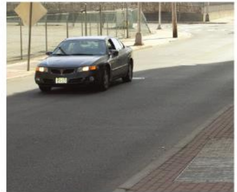
Missing truncated domes at Essex Avenue & Main Street intersection; severely faded crosswalk markings.
