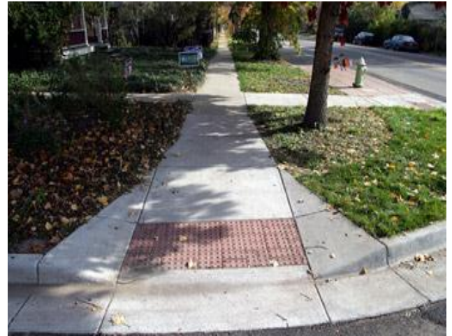
ADA Compliant Curb Ramps
