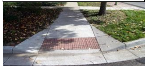
ADA Compliant Curb Ramp
