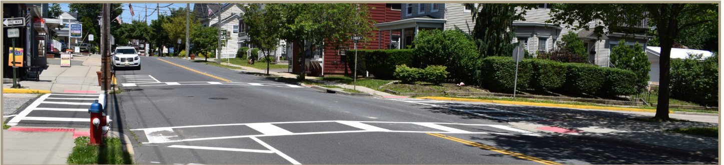
Figure 48. Demonstration project at the intersection of Church Street and Main Street, looking northwest.
