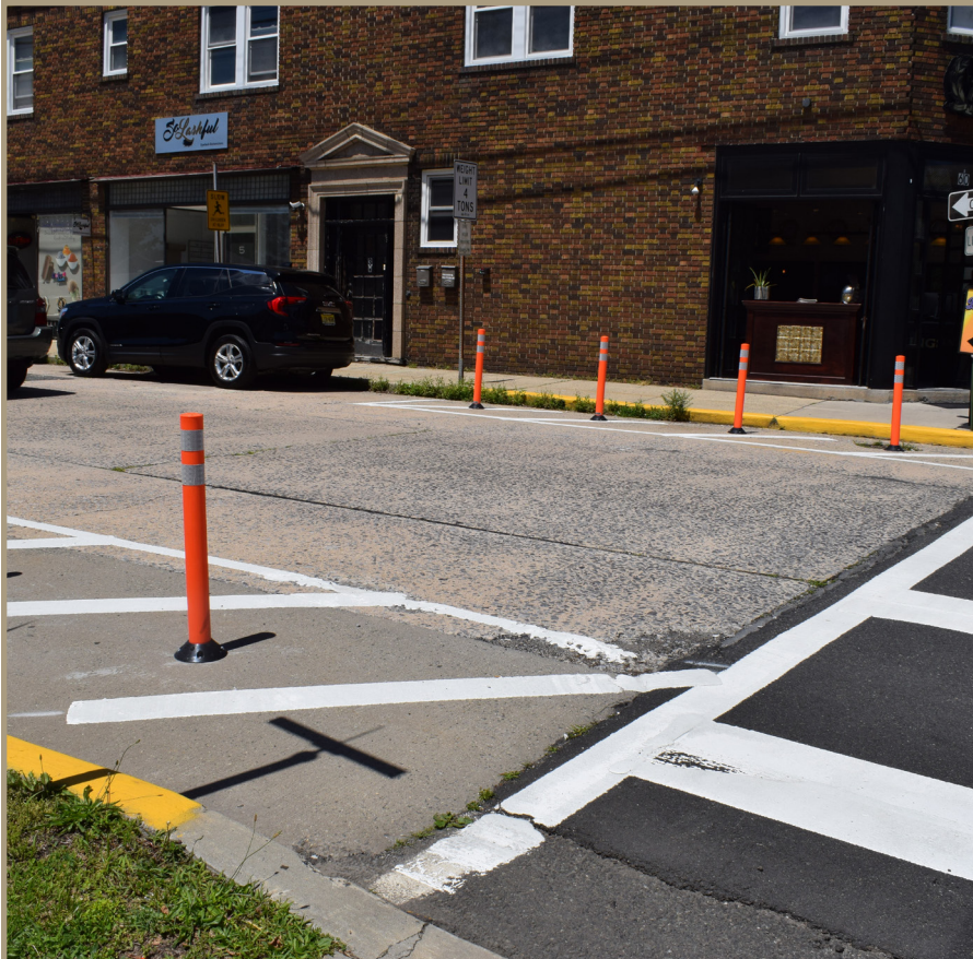
Figure 38. Plastic bollards and paint reinforce no parking near the intersection, looking southwest.
