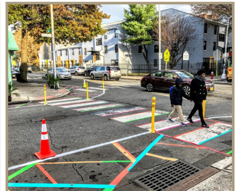
Figure 30. Demonstration paint, plastic bollards. Jersey City, New Jersey.
