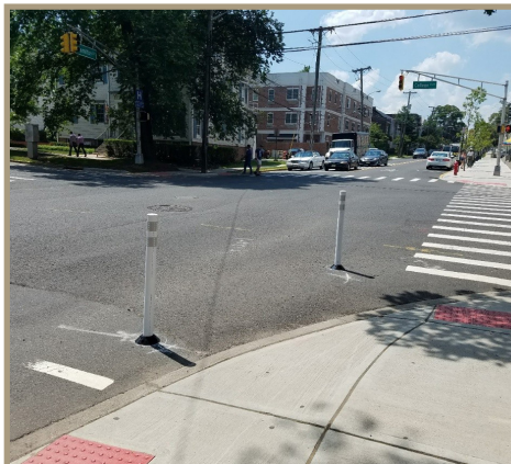
Figure 26. White plastic bollards to alter turning radius. New Brunswick, New Jersey.
