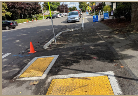
Figure 31. Sidewalk built using parking stops, Seattle, Washington.
