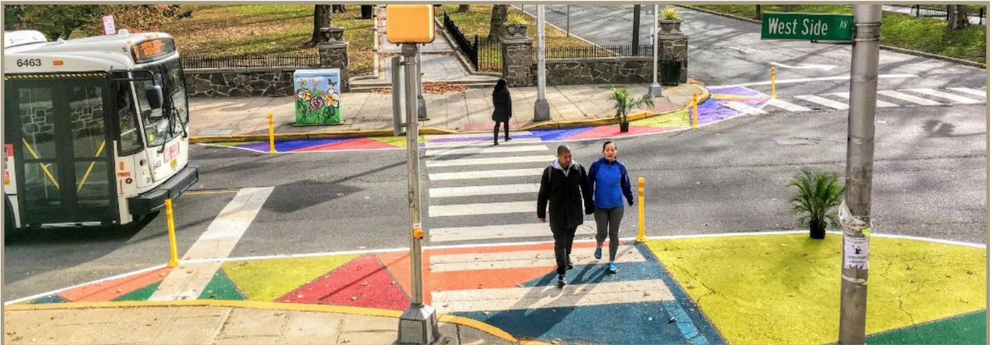
Figure 17. Painted curb extension in Jersey City (Photo credit: Street Plans)
