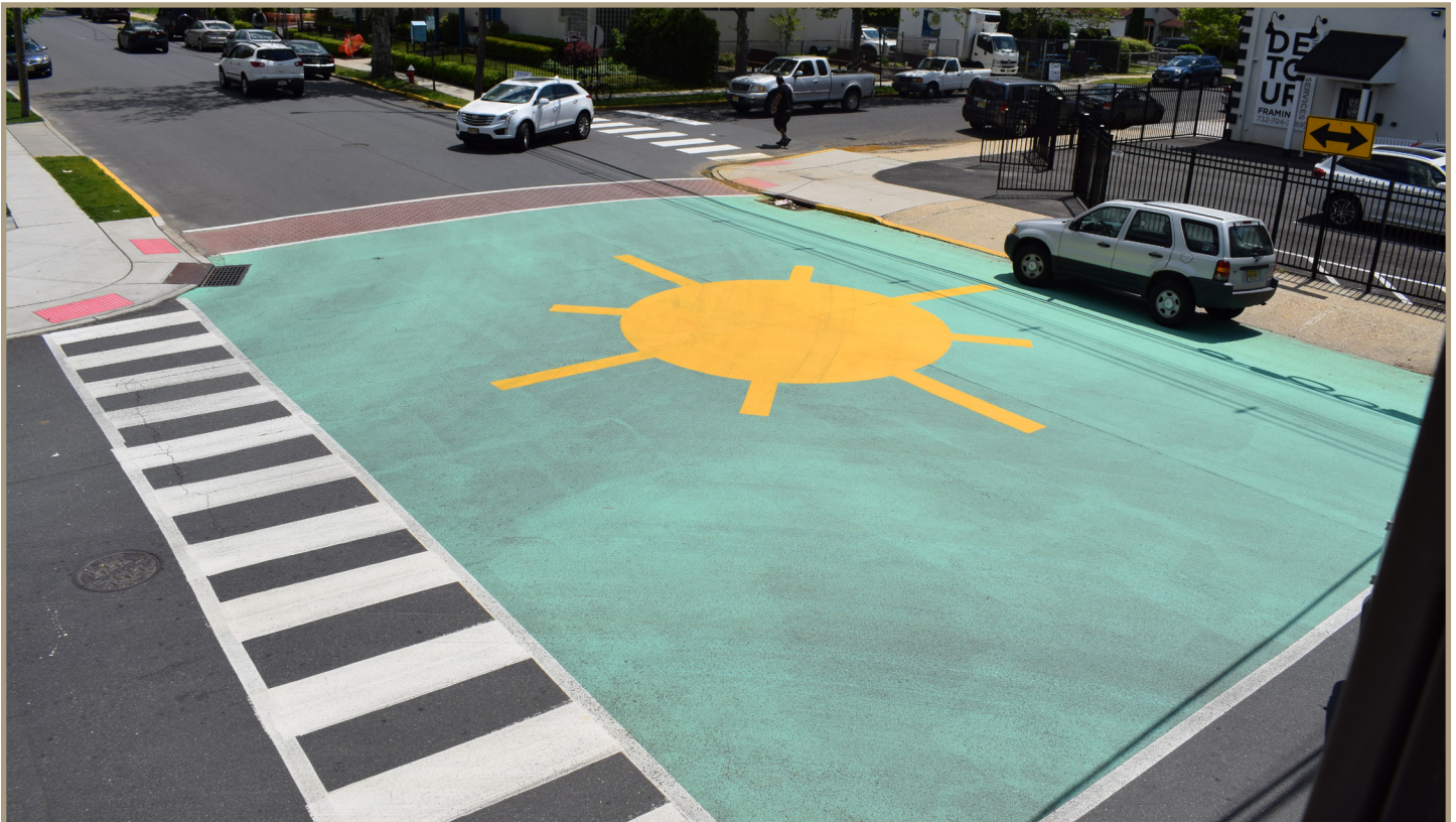
Figure 46. Intersection mural installed in Red Bank, New Jersey encourages drivers to look out for pedestrians.
