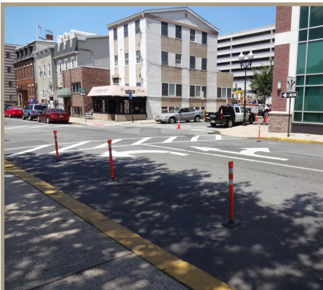
Figure 25. Orange plastic bollards to prevent illegal parking before intersection. New Brunswick, New Jersey.
