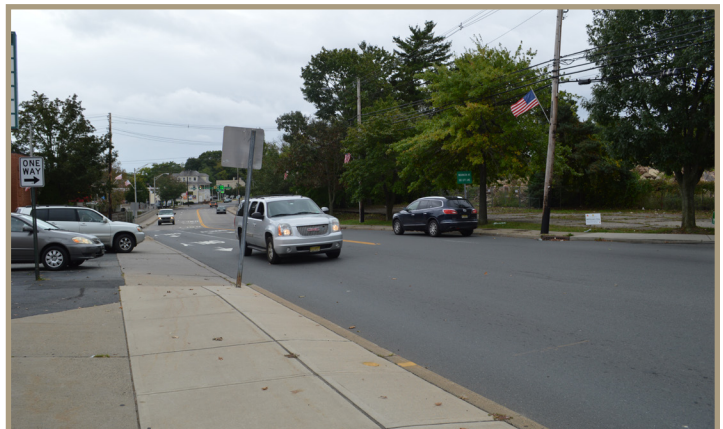
Figure 21. Main Street expands into four lanes south of the Ford Avenue intersection, looking southeast on Main Street (photo taken before installation).
