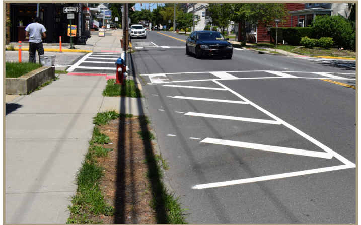
Figure 4. The installed improvements at the intersection of Church Street and Main Street, looking northwest.
