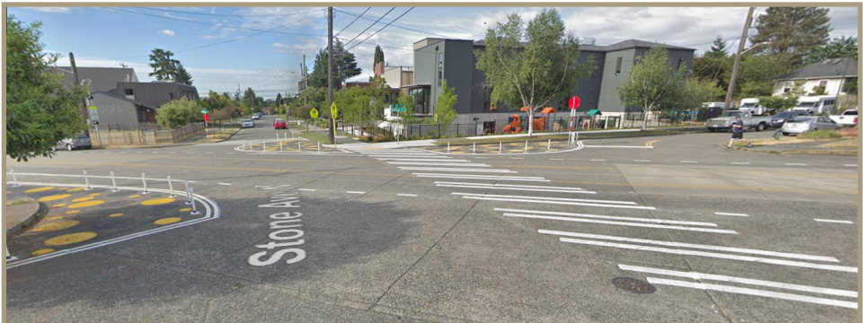
Figure 32. Street realignment with white plastic bollards, paint. Seattle, Washington.
