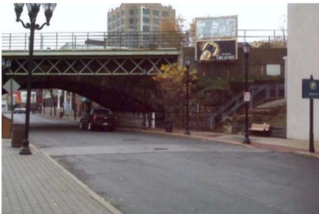
Figure 16 Current Grand Street Mid-Block Crosswalk
