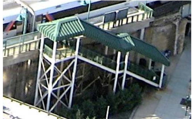
Figure 29 Covered Stairway at Station
