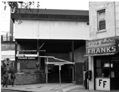
Figure 5 Main Entrance to Elizabeth Station
