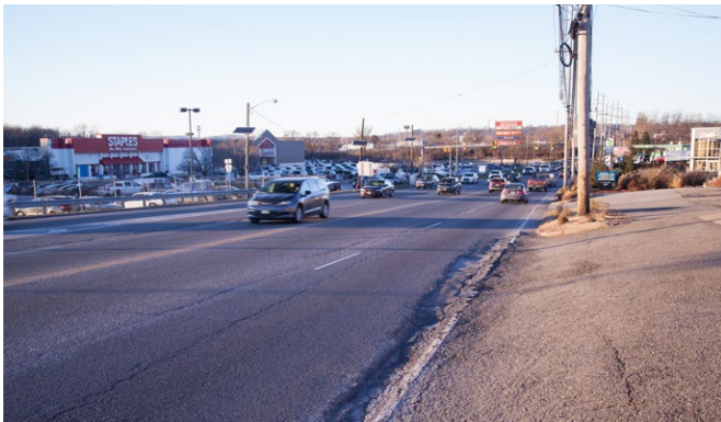
Fig.12. Riverview Drive - Totowa, Passaic County
