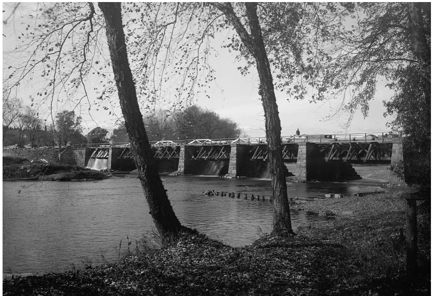
Fig.34. Pompton River Aqueduct near Lincoln Park-Wayne border Credit: Library of Congress, Prints & Photographs Division, LC-DIG-det-4a07257v
