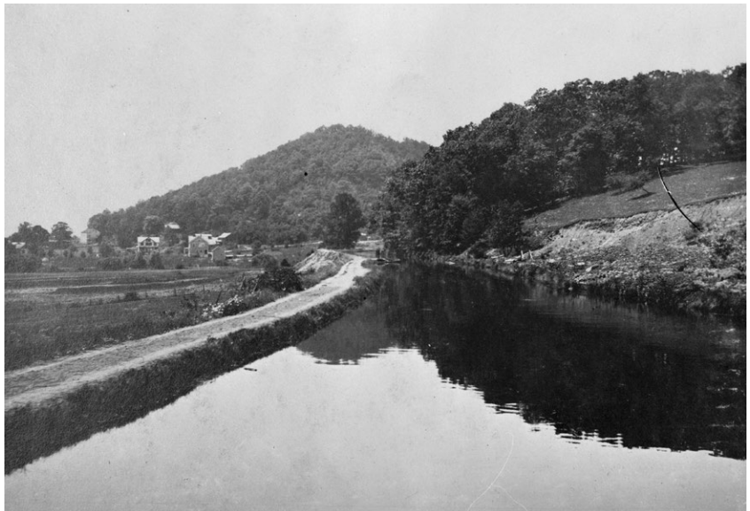
Fig.38. Canal prism looking west toward Hackettstown
