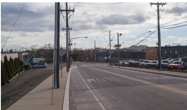
Fig.7. Linden Avenue - Jersey City, Hudson County
