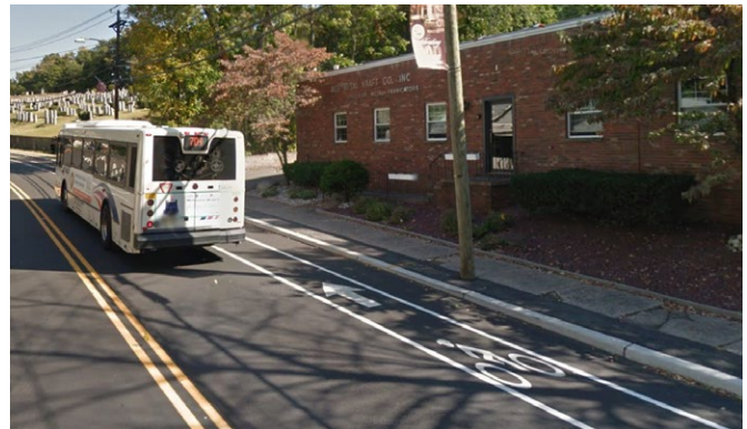
Fig.30. Existing: McBride Avenue, Woodland Park, Passaic Co.
