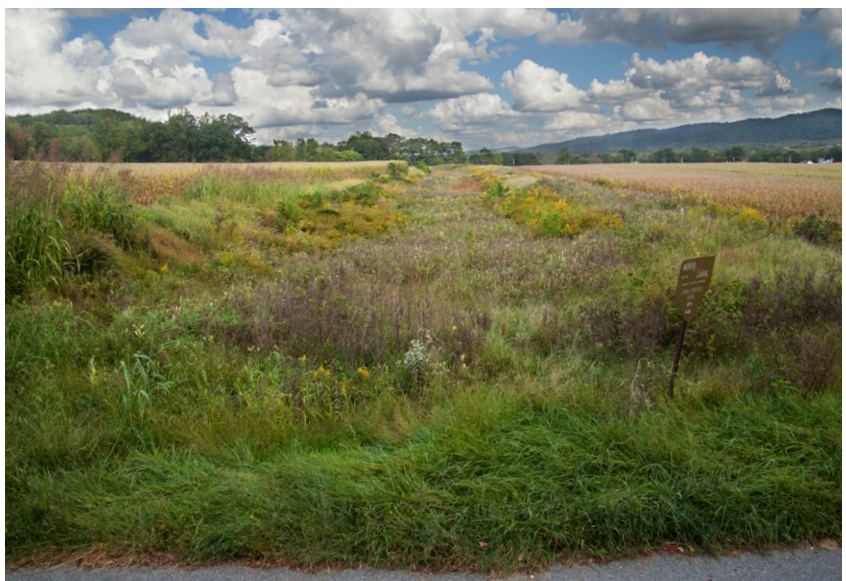
Fig.39. Canal prism at Whites Road, Warren County
