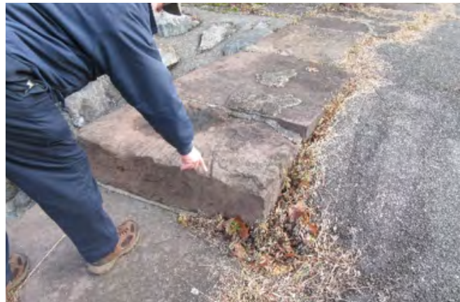
Grooves in the stone along a lock beside the Musconetcong River were made by the ropes pulled by mules as they moved canal boats into position. Such authentic features evoke a deep sense of time and history.
