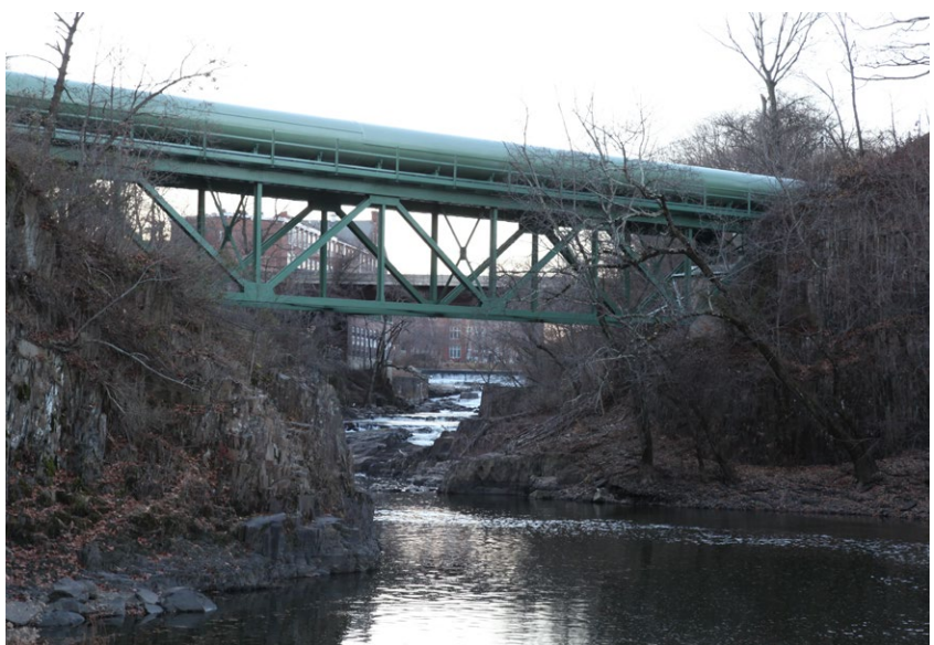
Fig.35. Site of former aqueduct in Little Falls, Passaic County
