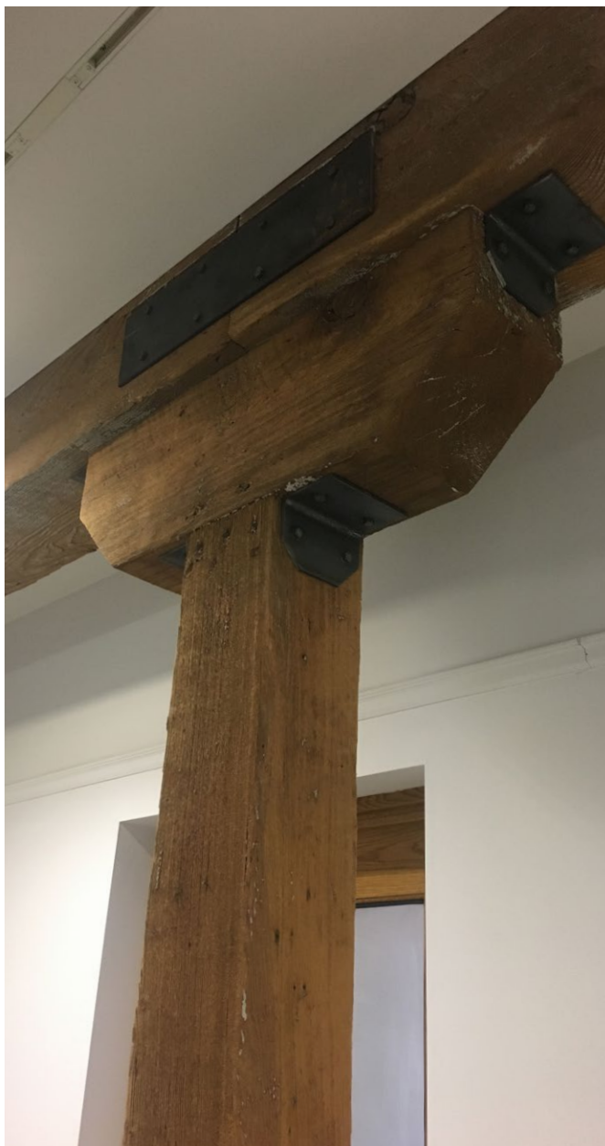
Fig.55. Wooden Posts & Galvanized Steel Hardware
