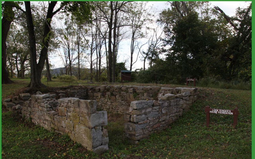
Fig.47. Lock tender's house foundation, Bread Lock Park, Warren County
