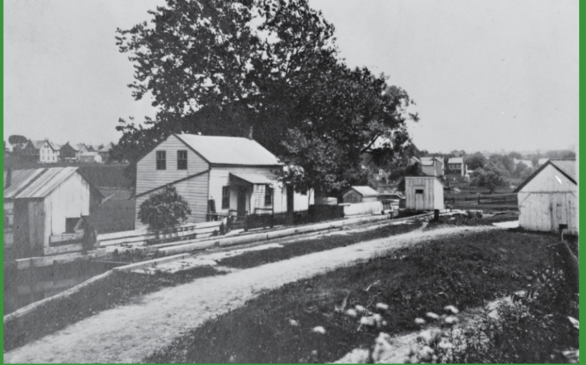
Fig.46. Lock tender's house at Lock 8 West
