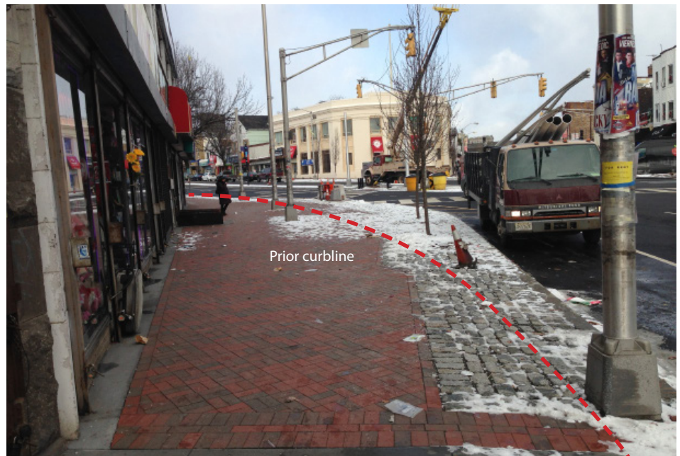
On Bloomfield Avenue, one dedicated turning lane was eliminated and the corner radius was reduced in order to provide a larger pedestrian area, calm traffic and reduce crossing distances.
