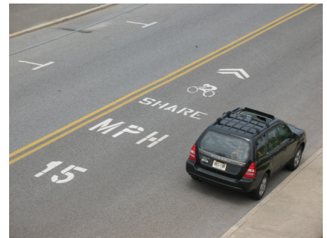
This bicycle boulevard on Haven Avenue in Ocean City gives priority to bicyclists with a low speed limit and large road markings.
