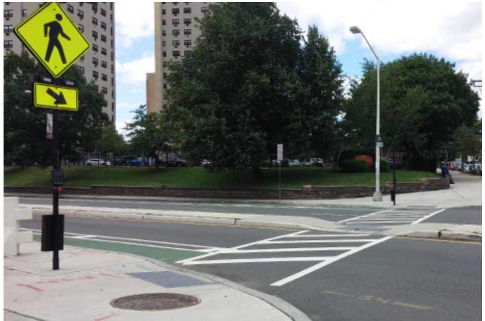
Rectangular rapid flashing beacon shown at West Market Street and Littleton Avenue.
