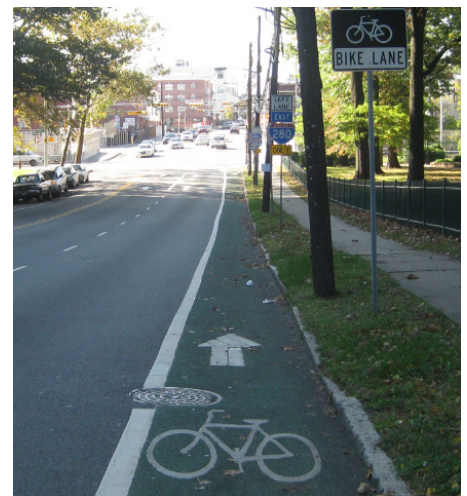
A curbside bike lane and signage on Clifton Avenue.
