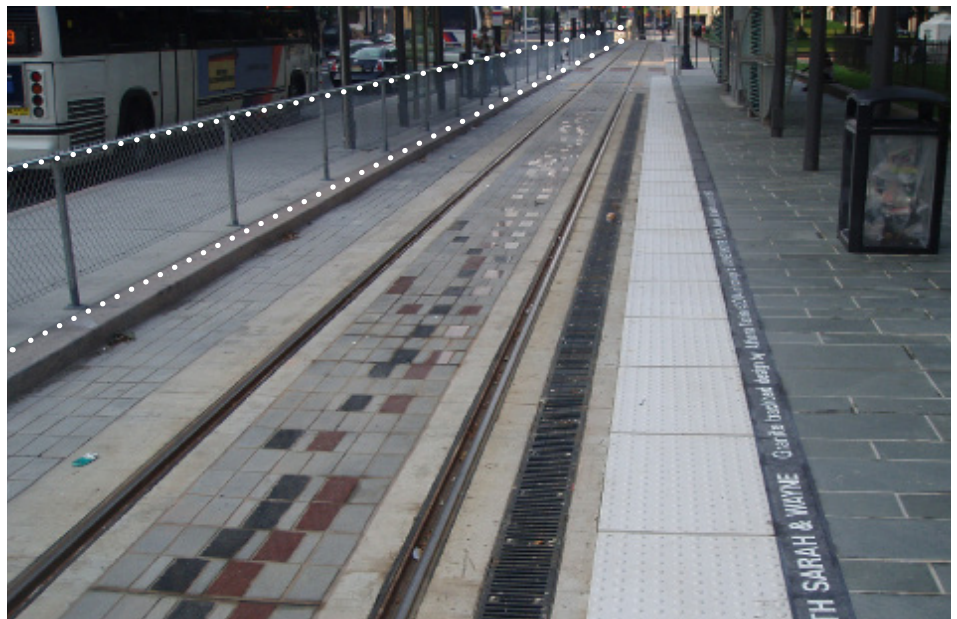
Pedestrian fences at rail stations to prevent pedestrian from crossing the tracks.
