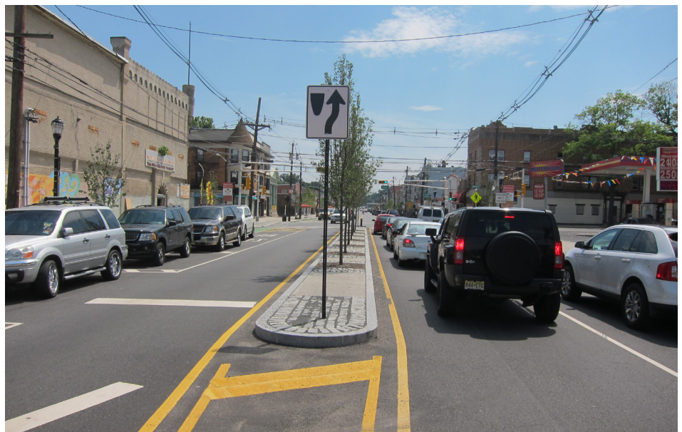
Gateway treatment on Mt. Prospect Avenue entering the Forest Hill neighborhood.
