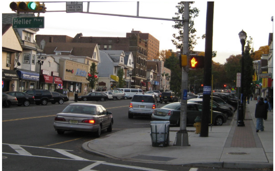
Curb extensions on Mt. Prospect Avenue significantly reduce the crossing distance by extending the sidewalk into the angled parking lane.
