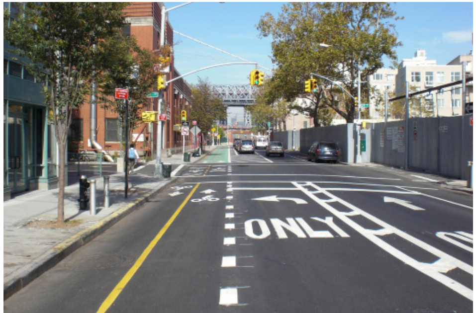
A mixing zone for vehicles turning left on to S 9th Street from Kent Avenue across the separated bicycle lane. The bicycle lane has its own traffic signal.
