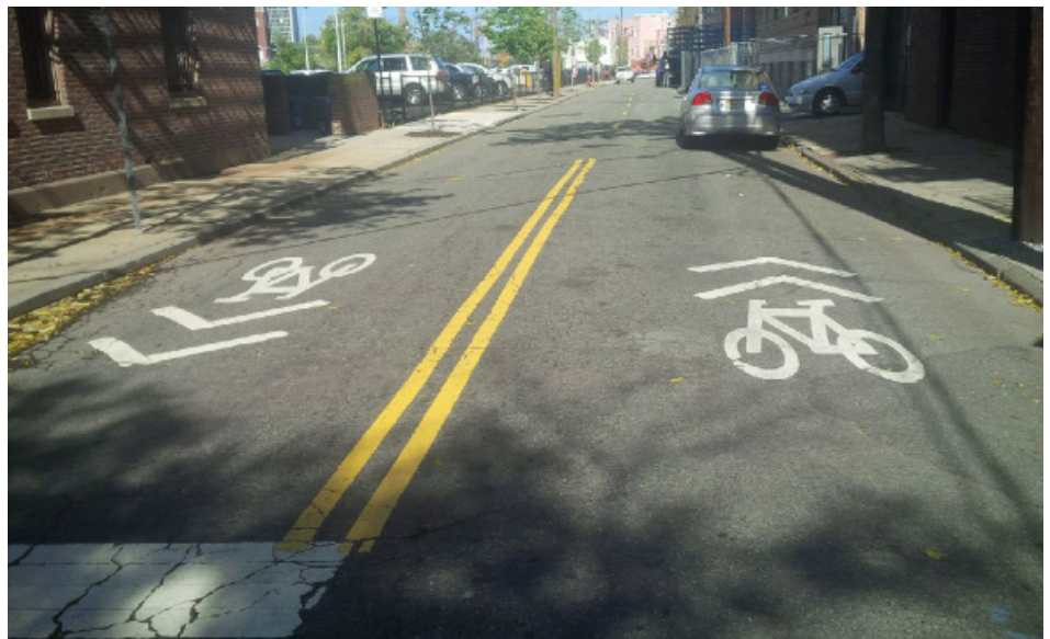
A sharrow indicates a shared roadway on a narrow, two-way street, Essex Street.
