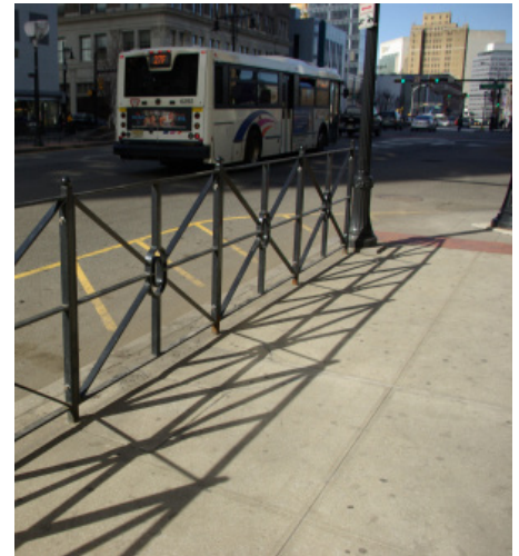
Pedestrian fences on the corner of Broad Street and Raymond Boulevard guide pedestrians to the
