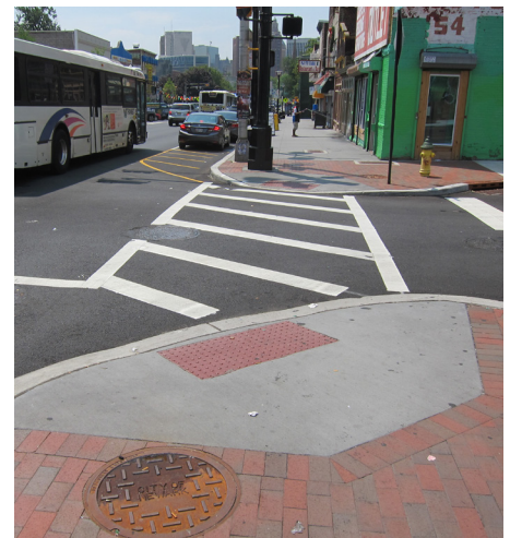
Broadway and Crane Street concrete curb ramp with brick edge.
