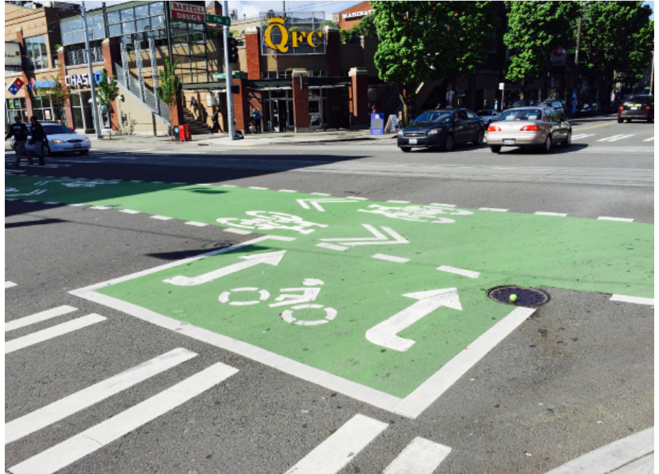
A two-stage turn queue box on Broadway in Seattle gives bicyclists a safe place to wait for a green light to turn across Broadway and onto Pike Street.
