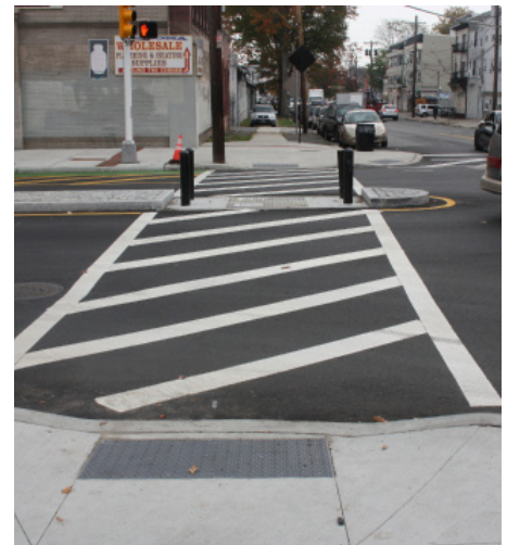
Pedestrian refuge island on Mt. Prospect Avenue at intersection of Verone Avenue.
