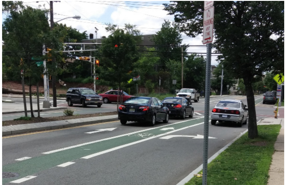
Irvine Turner Boulevard was converted from two lanes per direction to one lane per direction with a bike lane, a median and left-turn lanes at intersections.
