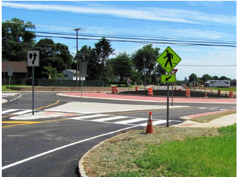
A roundabout in Burlington County, NJ calms traffic and provides safe crossings for pedestrians.
