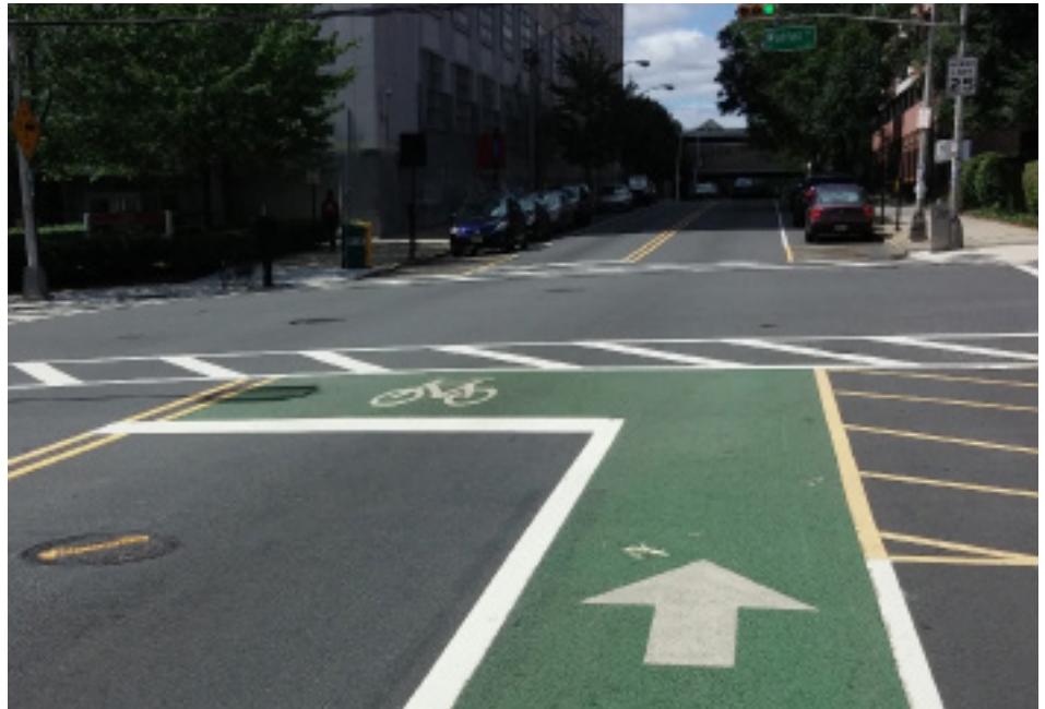
This bike box, located on the Rutgers University Campus, creates space for bicyclists to make a left turn to head east on Warren Street.
