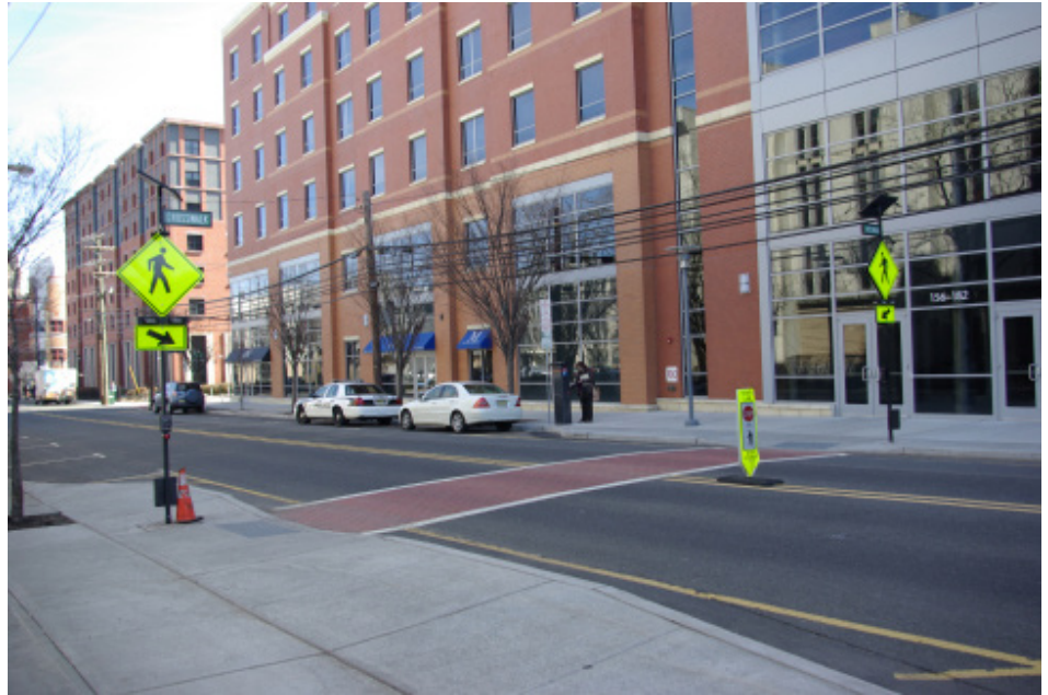
LED light panels located above the arrow will flash when the push-button is activated by a pedestrian, Warren Street.
