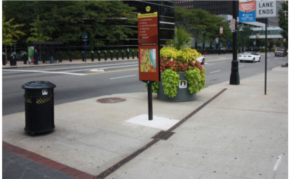
Curb extension at Market Street and Mulberry Street.
