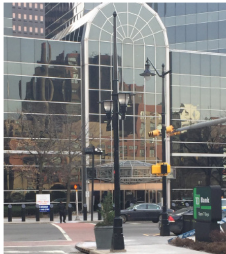
Pedestrian-scale double-head fixture on Mulberry Street.
