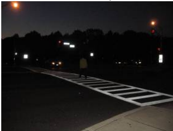
Photo C: North crosswalk of intersection
