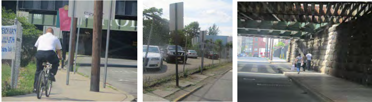
Improperly placed sign poles, sidewalks in poor condition and dark underpasses are not conducive to a safe and pleasant walking experience.
