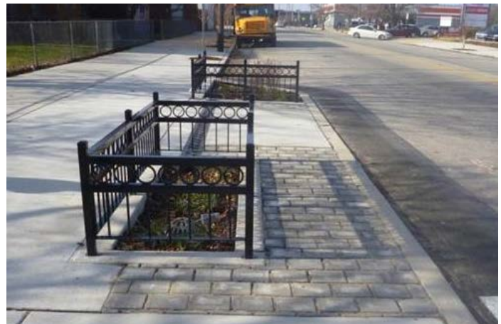
Stormwater Curb Extension; Philadelphia, Pennsylvania
