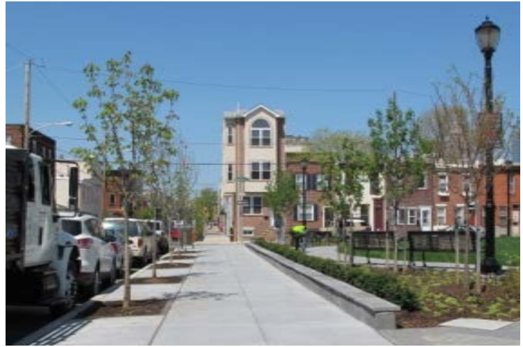
Infiltration Trench; Julian Abele Park, Philadelphia, Pennsylvania
