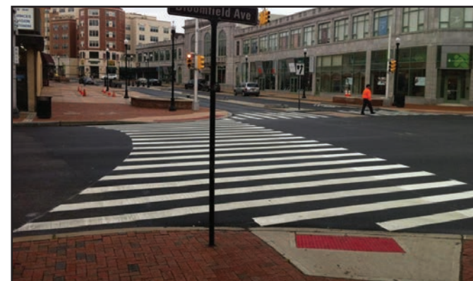
This High-Visibility Ergonomic Crosswalk Follows Pedestrian Desire Lines in Montclair, New Jersey
