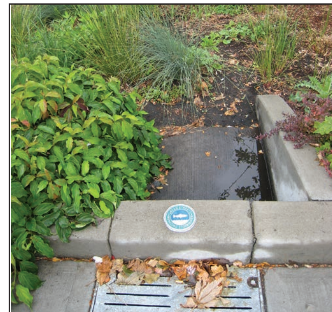
Storm Drain Outfall to Rain Garden
