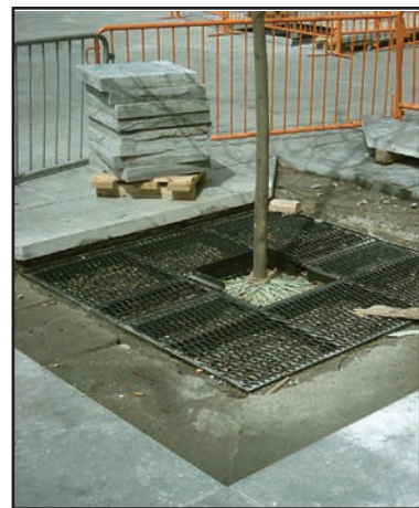
Paver Grate Suspension System Without Pavers Installed
