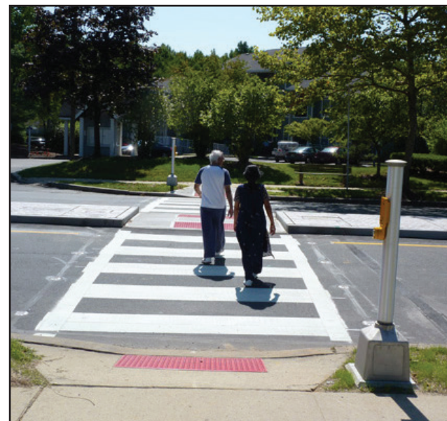
Pedestrian Refuge Island in West Windsor, New Jersey
