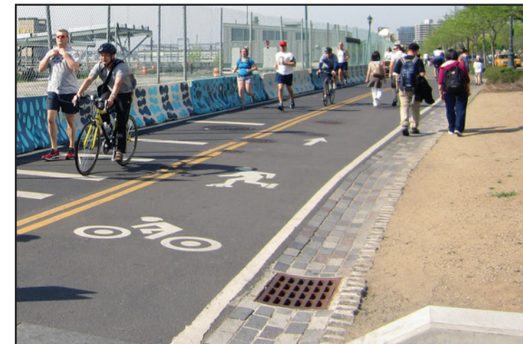
A painted concrete barrier is used along one edge and pavers form the other in this stretch of the Hudson River Greenway, NYC
