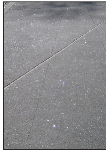
Tinted Concrete Pavement with Silica Carbide to Create Sparkle Effect
