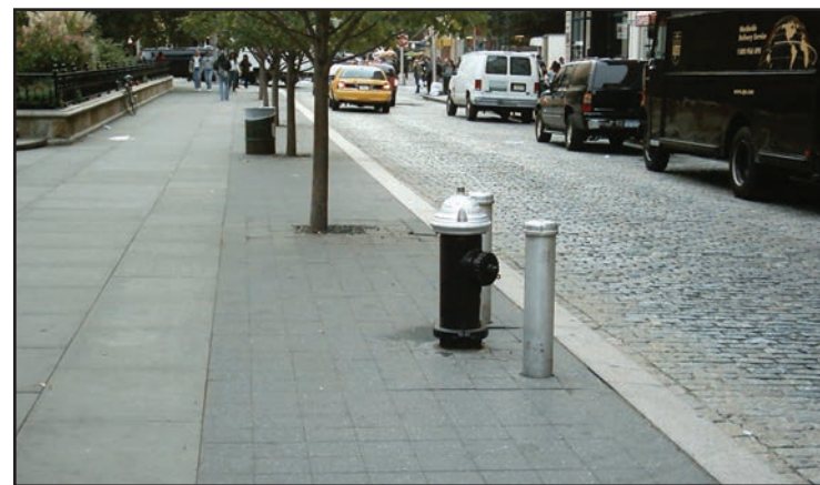
Decorative Pavement Materials (bluestone paving and square asphalt pavers on the sidewalk, extra wide granite curb and granite block in the road bed). Street Trees Utilize Paver Grate Suspension System.
