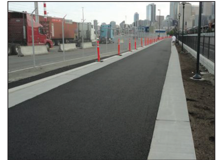
Asphalt Shared Use Path with Concrete Edging, Seattle, Washington
