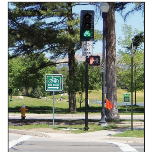
Bicycle Signals are Used to Provide Guidance for Bicyclists at Intersections Where They May Have Different Needs from Other Road Users (e.g., bicycle only movements, leading bicycle intervals), Salt Lake City, Utah
