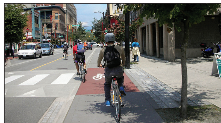
Colored Pavement and Variations in Materials are Used to Define Conflict Areas along the Carrall Street Greenway in Vancouver, British Columbia..
