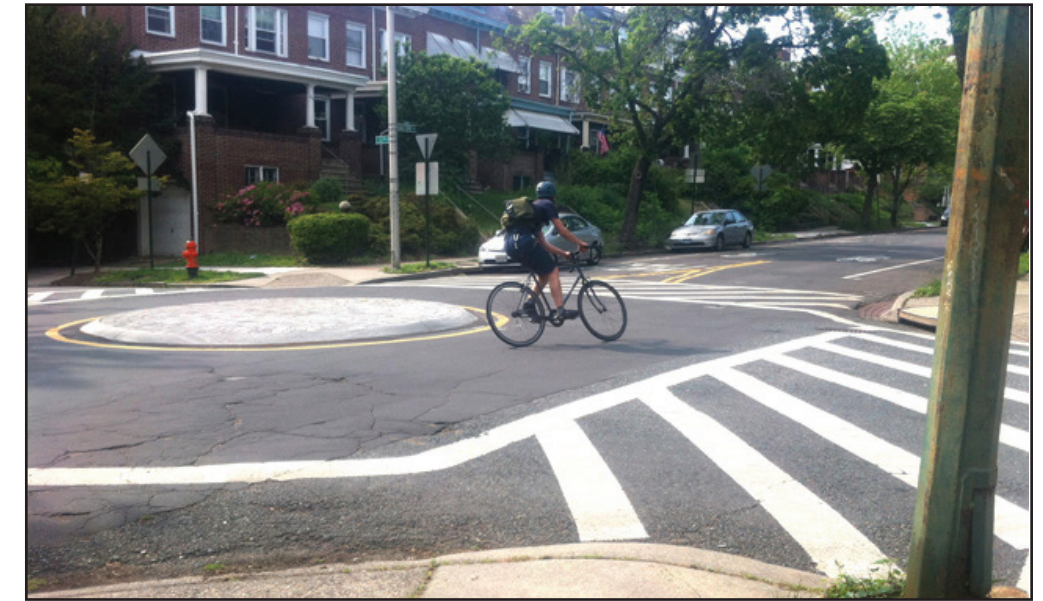
A Mini Traffic Circle on the Guilford Avenue Bicycle Boulevard Reduces Speeds and User Conflict, Baltimore, Maryland
