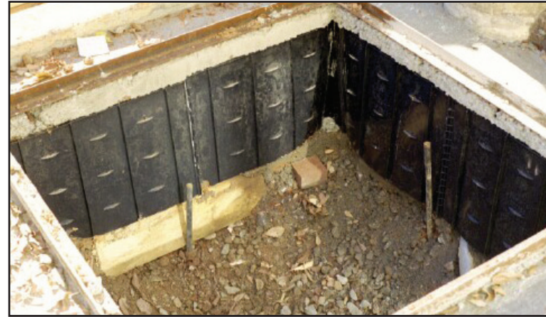
Root Barriers Prevent the Roots from Lifting the Sidewalk or Path but Curtail Growth
