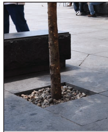
Paver Grate Suspension System with Pavers Installed
