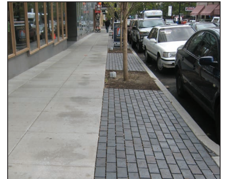
Porous Paver Amenity Strip
