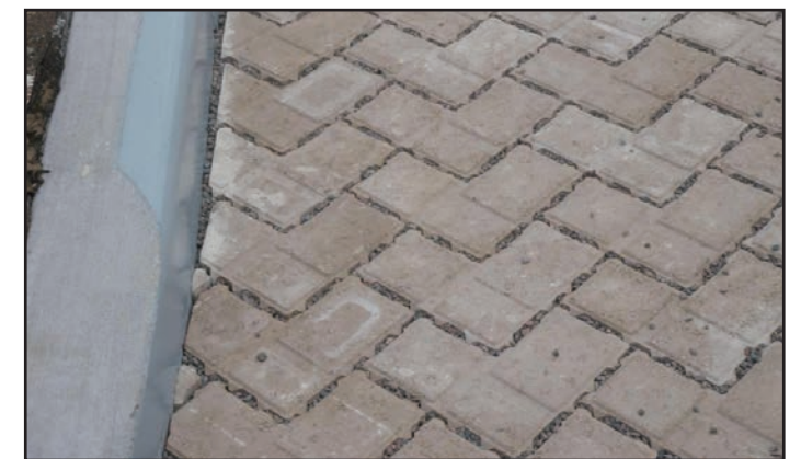
Porous Pavers in Parking Lot
