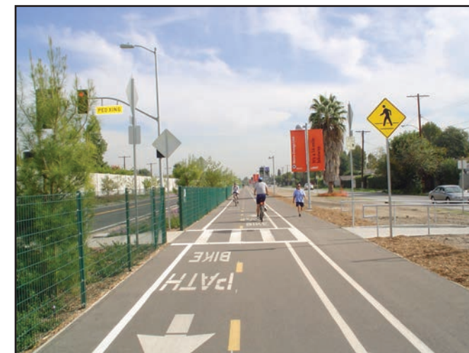
Striping and Pavement Markings are Used to Delineate Uses and Direction along The Orange Line Path, Los Angeles
