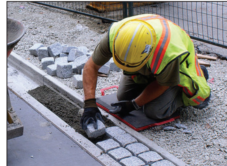
Paver Edge being Installed along Carrall Street Greenway, Vancouver
