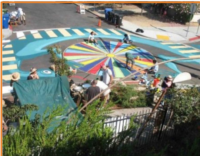
Decorative pavement markings on a neighborhood intersection
