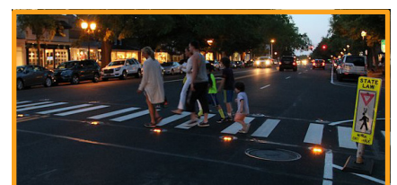
In-pavement crosswalk lighting
