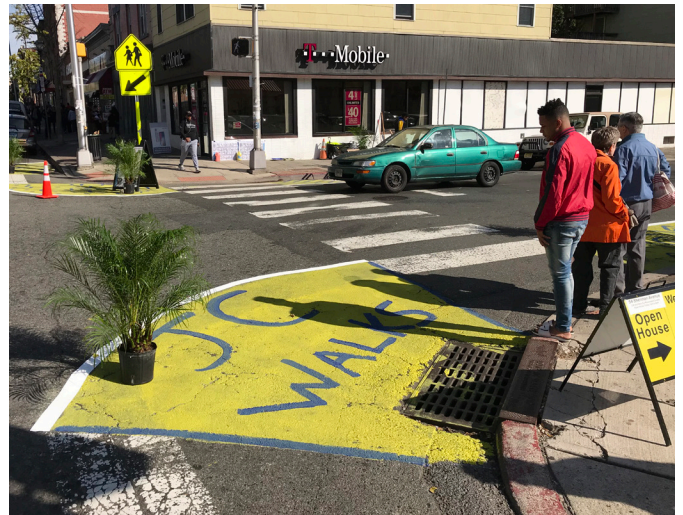
Painted curb extension and flexible delineators can be installed during the pilot project phase
