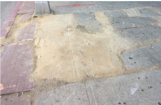
Inadequate sidewalk repair in the Heights
