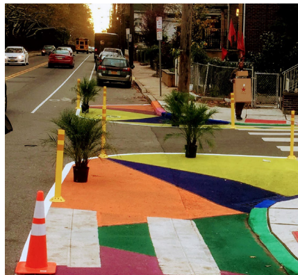
Painted curb extension and flexible delineators can be installed during the pilot project phase
