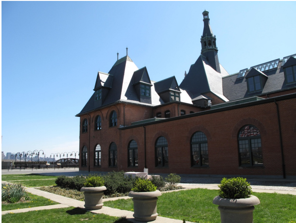
Figure 5-5 Historic CRRNJ Terminal
