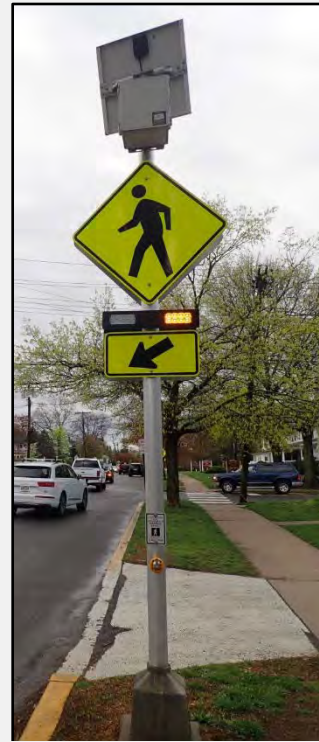
Rectangular Rapid Flashing Beacon
