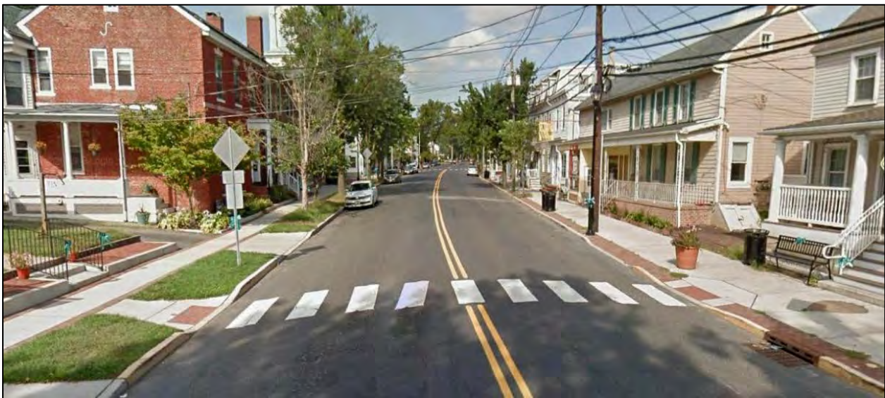
Figure 26 - Existing Mid-block Crosswalk with ADA Accommodation in Allentown
