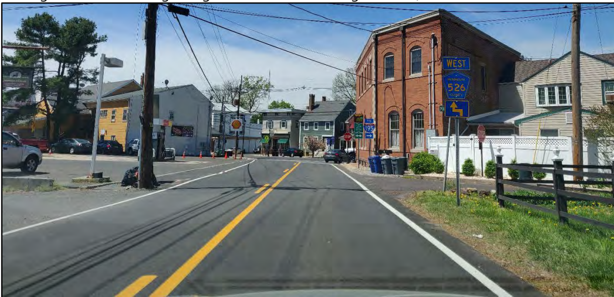
Figure 28: Missing Sidewalks on CR 526 Waker Avenue
