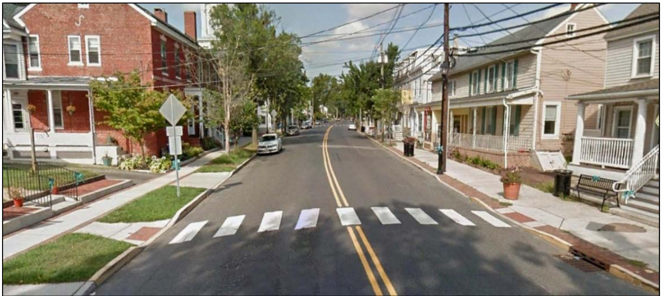
Figure 26 - Mid-block Crossing on CR524 (South Main Street)
