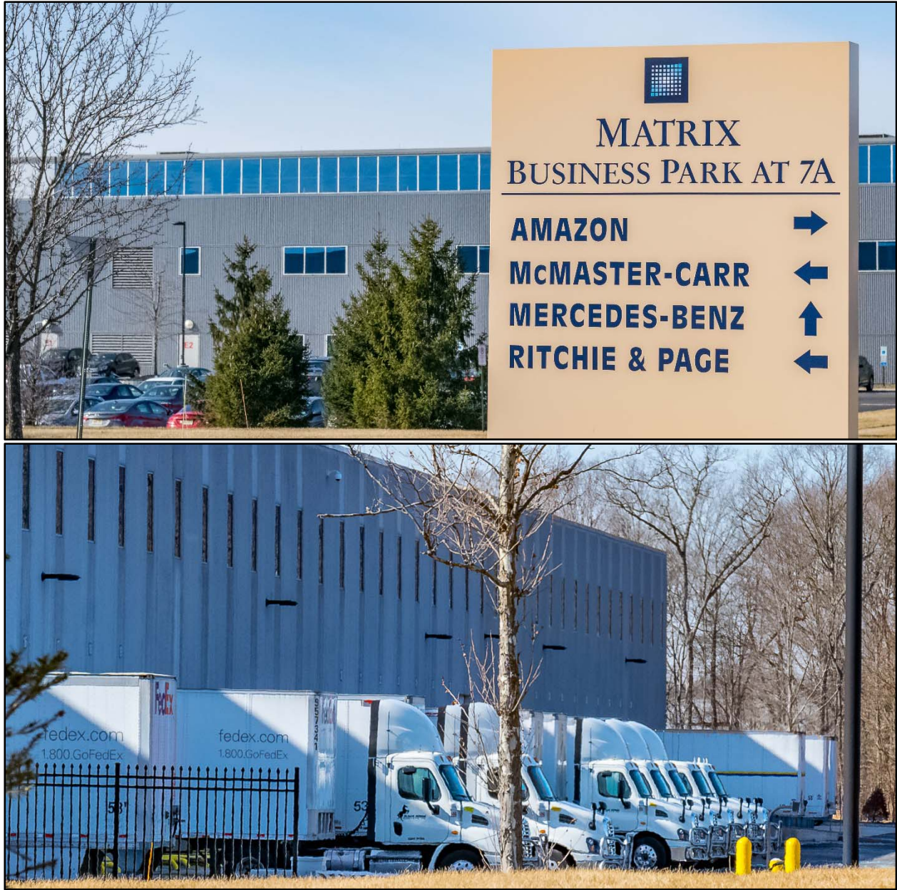
Figure 35 - Signage and Trucks at the Matrix Site
