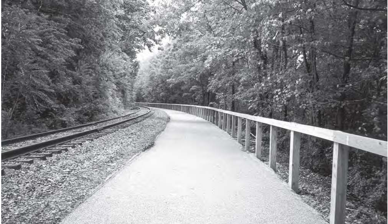
Sixty-one rails-with-trails now operate safely in the United States. For more information, see RAILS-WITH-TRAILS , by Rails-to-Trails Conservancy. Photo by Gwen Loose.
