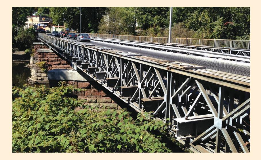
that have since deteriorated, leading to the bridge's classification as "fracture critical." The bridge is also classified as functionally obsolete due to substandard width and inspections have detected soil erosion around its piers and abutments. A 15 mph speed limit is posted for bridge traffic.
