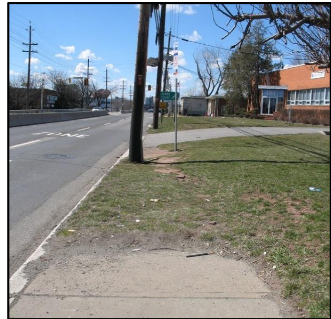
Lack of sidewalk connectivity
