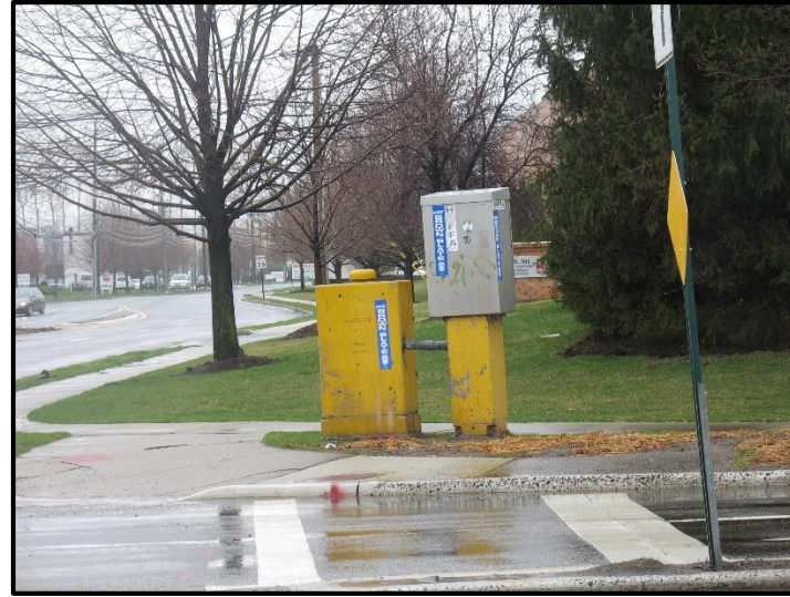
Antiquated signal controller
