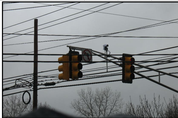
Utility wires block signals
