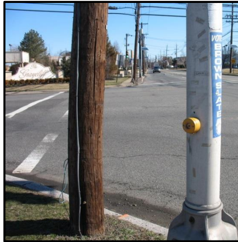
Pedestrian push button not adjacent to crosswalk
