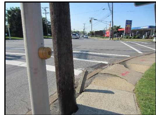
Push button not adjacent to crosswalk
