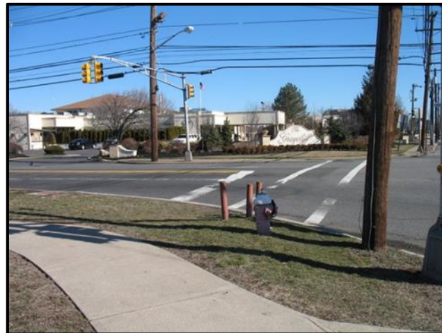
Lack of sidewalk connectivity
