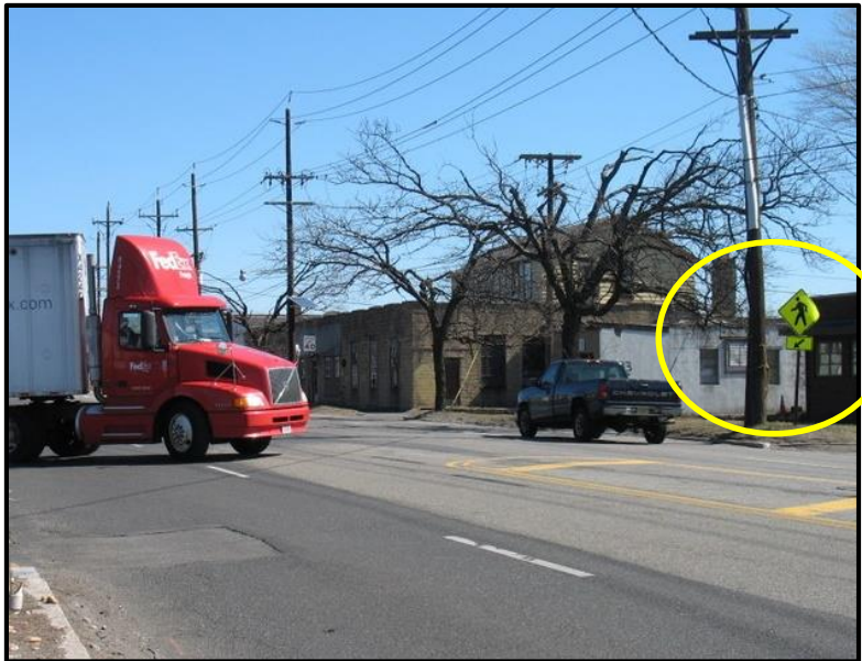
Lack of marked crosswalk (although signed)
