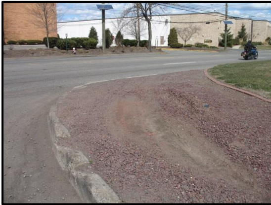
Damage from turning trucks
