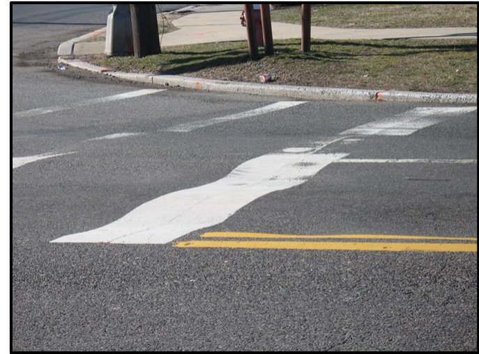
Worn crosswalk striping
