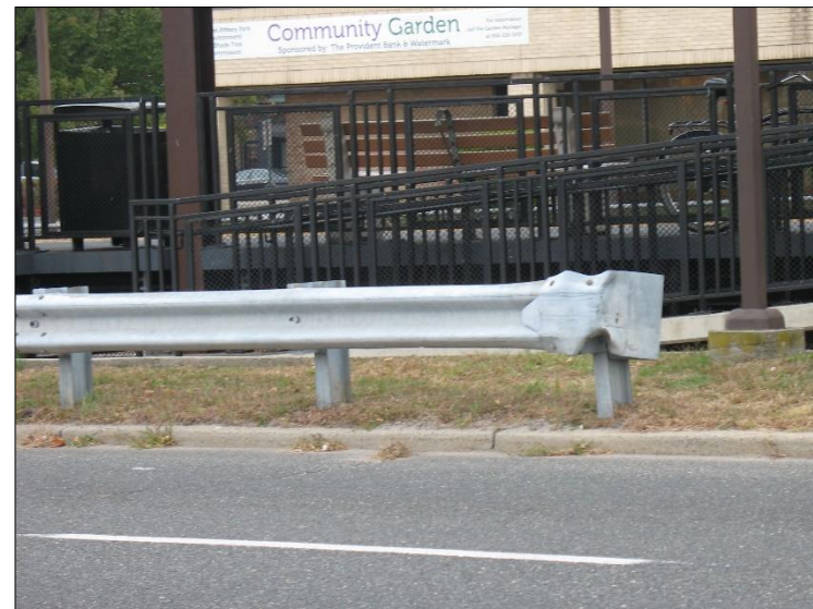
Figure 20 – Guide rail end treatment damaged
