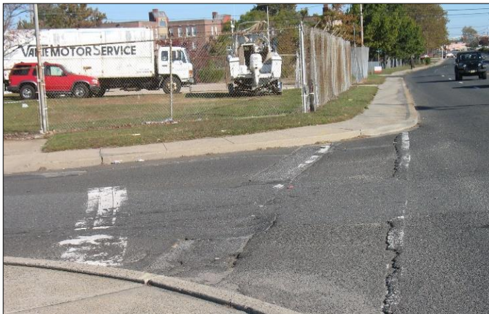
Figure 15 – Faded pavement markings
