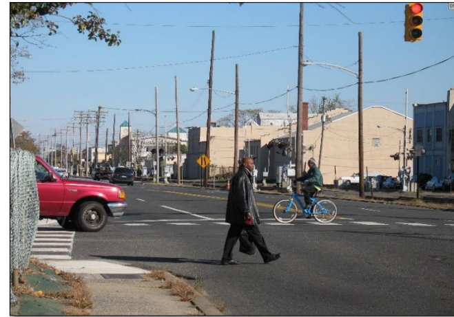
Figure 14 – Limited sight distance for southbound vehicles turning from Mattison Avenue
