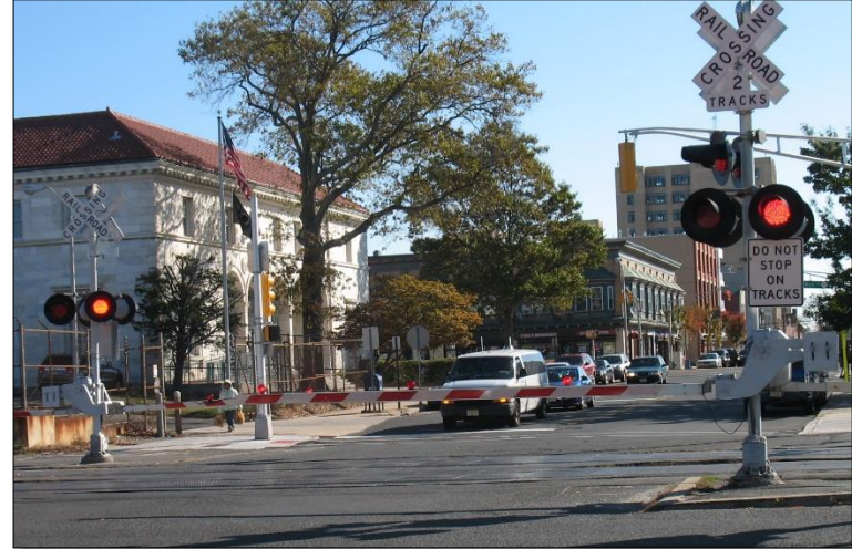
Figure 18 – Lack of pavement markings on railroad crossings
