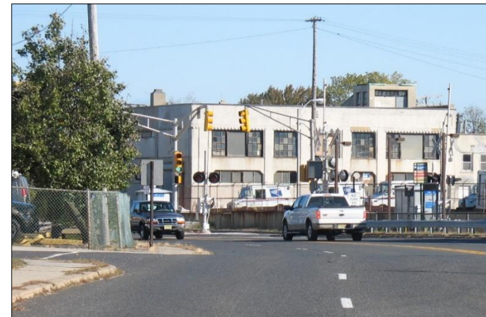
Figure 116 – Limited sight distance of southbound vehicles from Mattison Avenue
