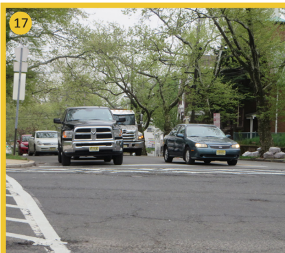
The vertical curve makes visibility of stop bar difficult.
