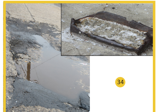
There are tripping hazards in the sidewalks on Lyons Avenue.
