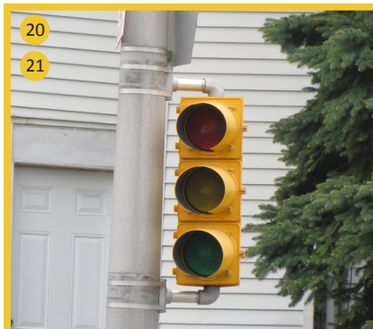
Traffic signal bulbs are not functional on 8-inch heads.
