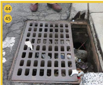
Inlet with curb piece missing and full of garbage.
