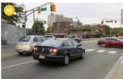
40 Negative offsets on the northbound and southbound approaches may be the reason for the high frequency of left-turn crashes
