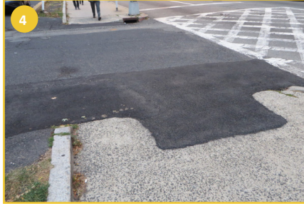
Uneven sidewalks at driveway entrances
