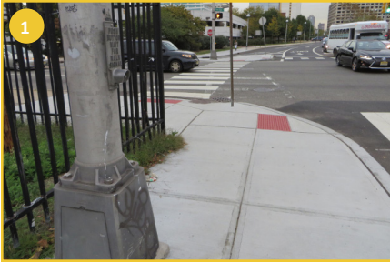
1 Push buttons are located far from intersection, and appear to be underutilized
