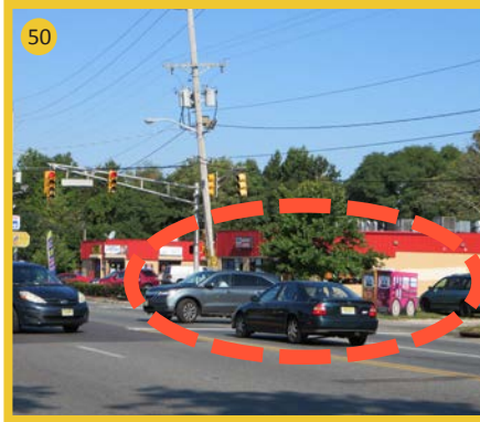
Driveway access on north side of intersection creates conflict
