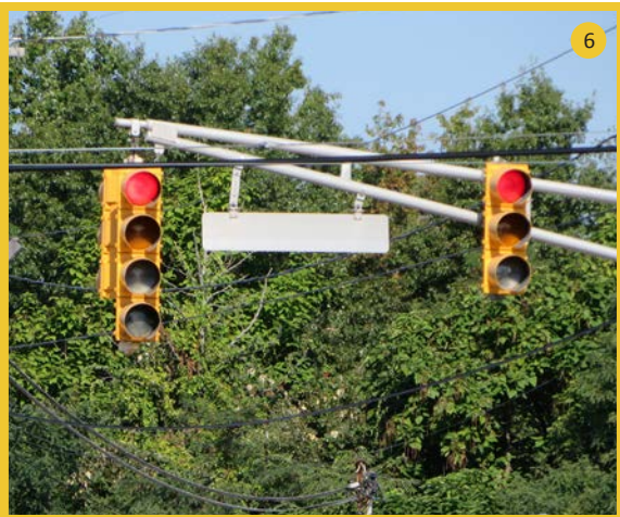
There are no retroreflective back plates
