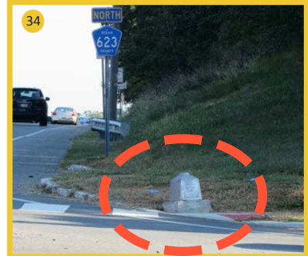
Pedestrian push button broken off from pedestal
