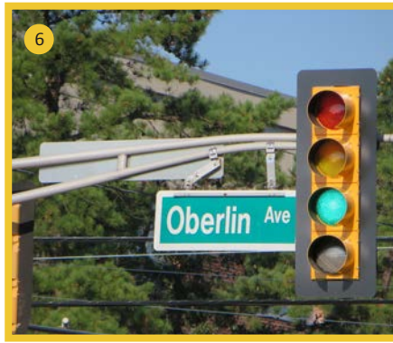
6 Backplates lacking retroreflective strips
