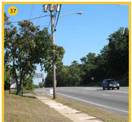
Crest of southbound New Hampshire Avenue
