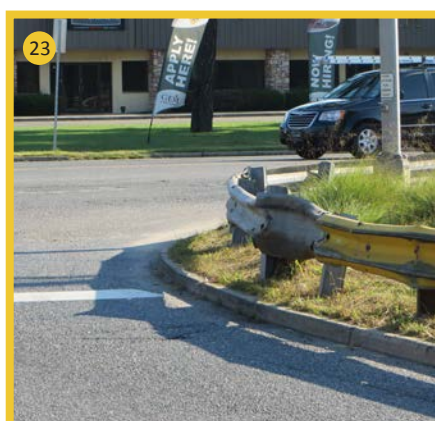
23 Damaged guiderail on southeast corner
