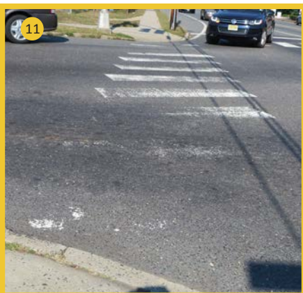
Faded pavement markings
