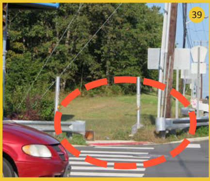
Guardrail not up to design standards
