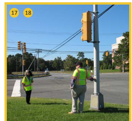
17 18 There are no pedestrian accommodations although there is a push button
