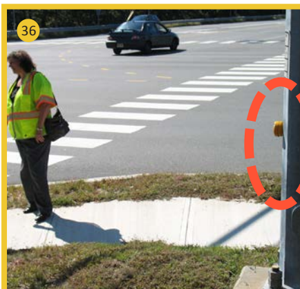
Pedestrian push button too far from ramp
