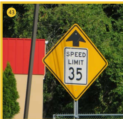
Speed limit stepdown not located prior to residential area
