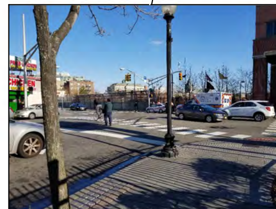
Many curb ramps were not ADA compliant.
