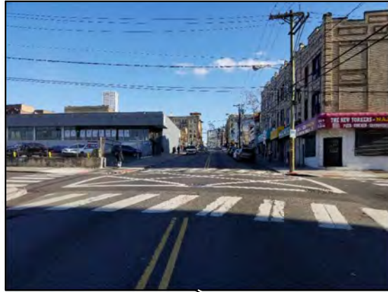
Curb heights along the roadway appear insufficient.
