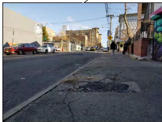
Sidewalks are in poor condition along Sip Avenue.
