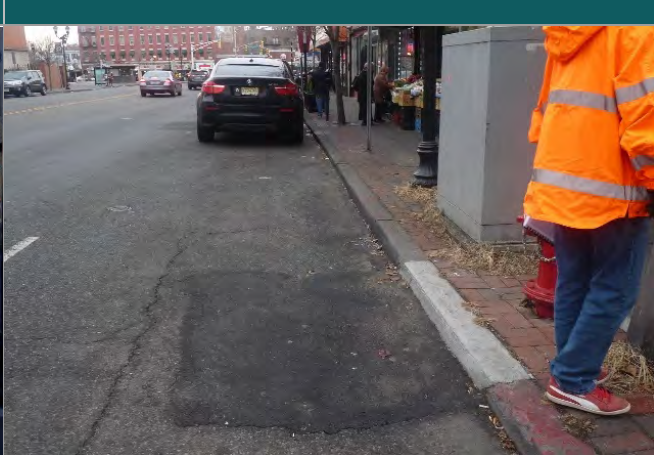
Pavement should be repaired in certain areas
