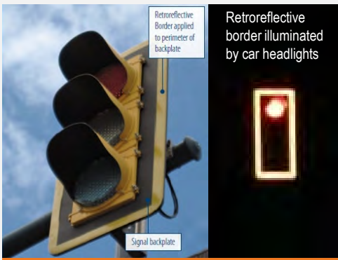
Backplates with Retroreflective Borders
