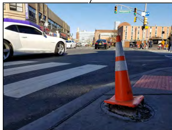
Signs are either improperly mounted or missing from multiple locations.
