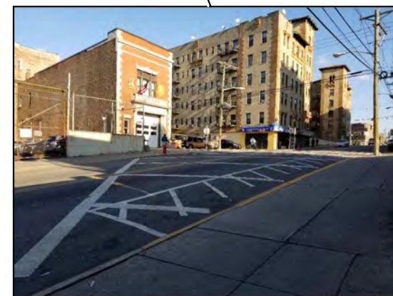
Irregular striping exists in front of the fire station.
