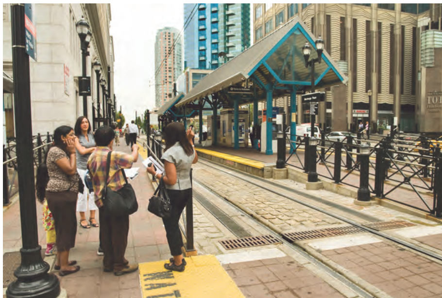
The future scenarios examined for Plan 2035 all forecast a significant increase in transit ridership. Light rail station, downtown Jersey City.
