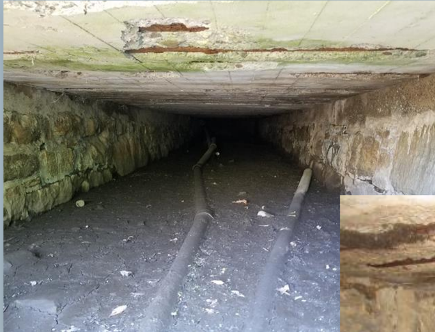
View Beneath Bridge
