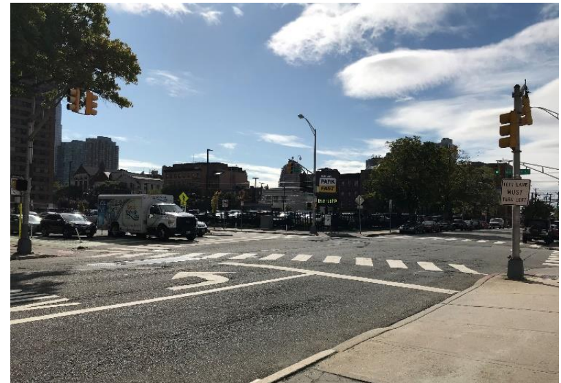
Skewed crosswalk increases pedestrian crossing distance
