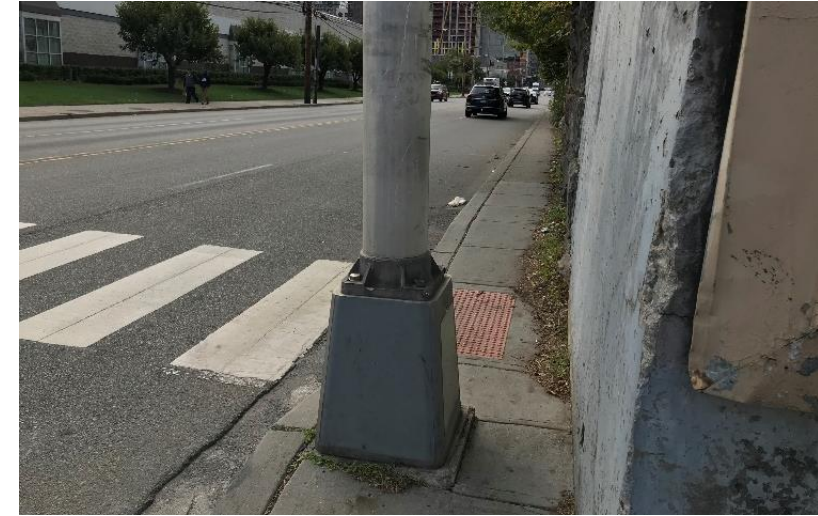
Sidewalk, curb ramp, and pushbuttons do not meet ADA compliance
