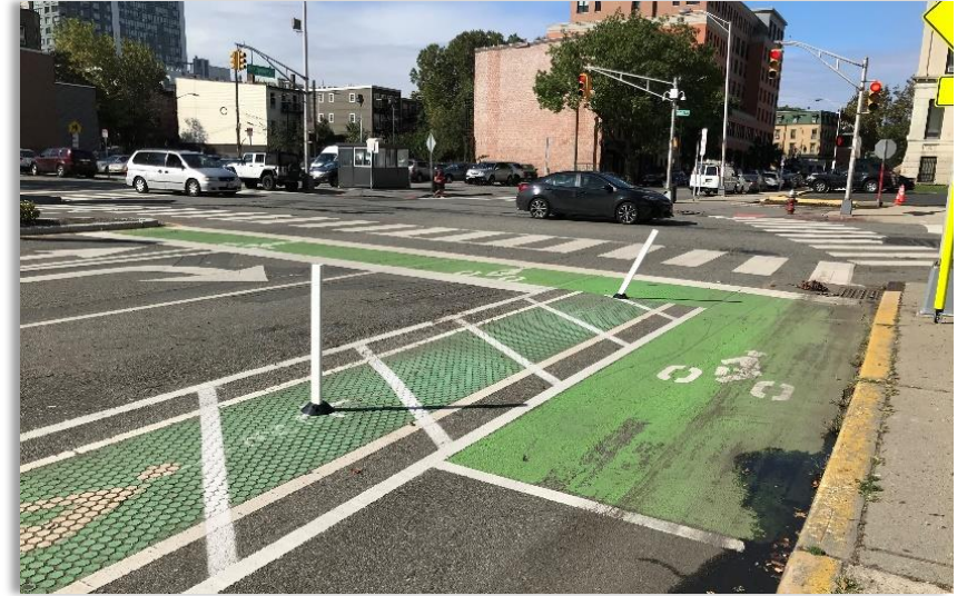
Buffered bike lane and bike box at Montgomery Street, looking west
