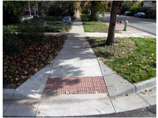
ADA Compliant Curb Ramps
