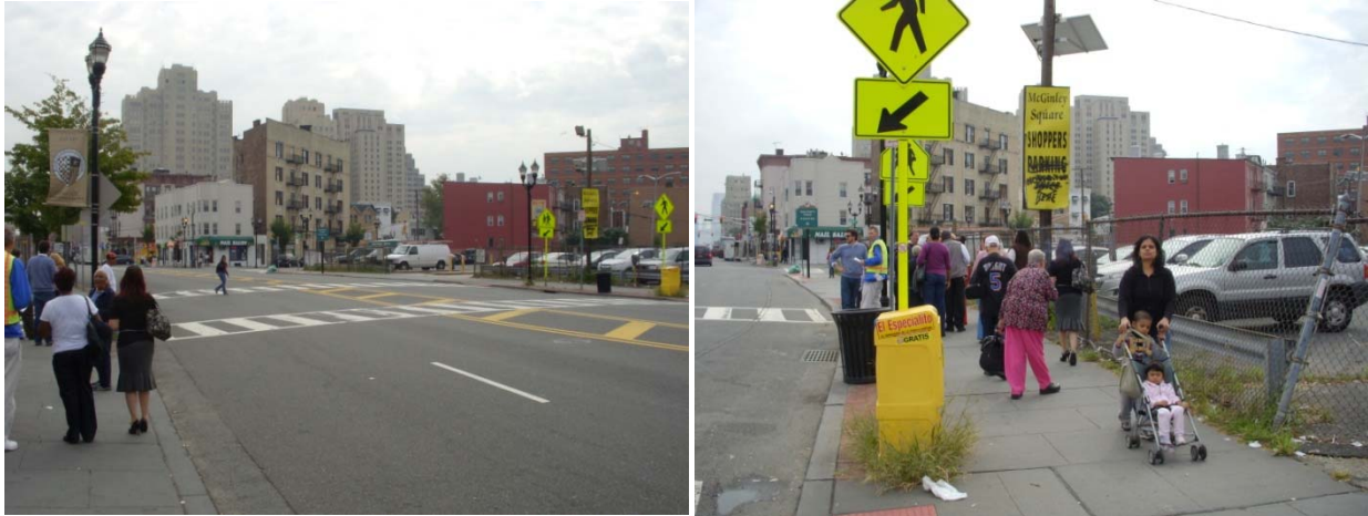
Issue Area – Pedestrian Safety: Signage & Median
