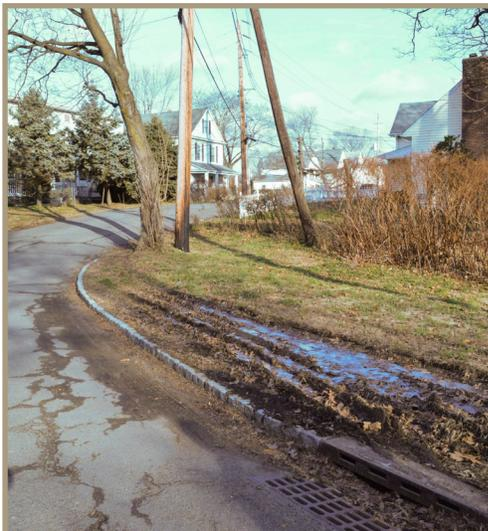
Figure 25. Tire tracks visible where drivers cut the curve.
