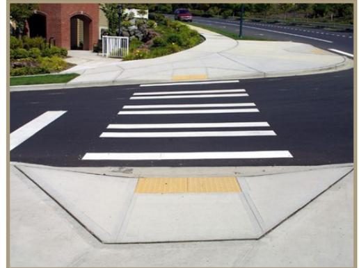
Figure 48. Curb ramps should direct pedestrians into the crosswalk.
