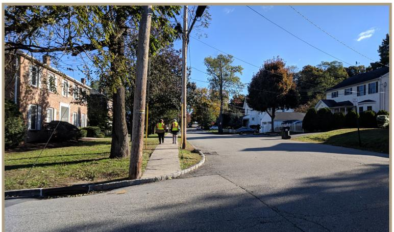
Figure 18. Sidewalk lacking wheelchair accessible ramp, and no painted crosswalks in any direction.
