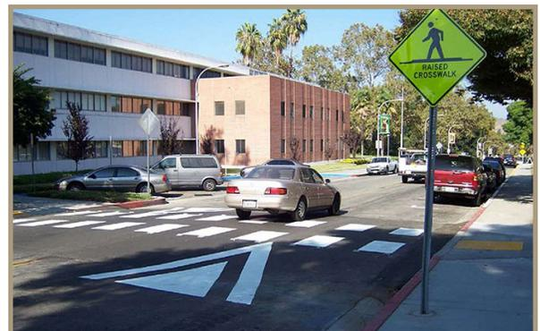
Figure 45. A speed table with a marked crosswalk (a raised crosswalk).
