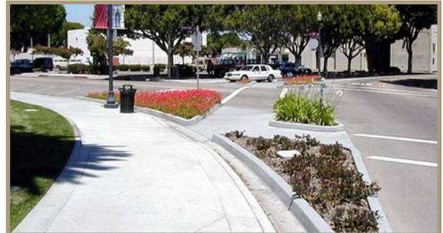
Figure 69. Curb extension design for reducing large turning radii. (Photo Credits: PBIC Image Library)
