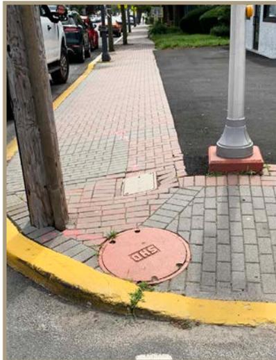
Figure 30. Uneven pavement near the Evergreen Avenue intersection.
