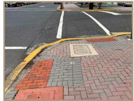
Figure 22. Curb ramps on Main Street at Fourth Avenue.
