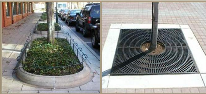
Figure 71. A curbed planting bed with a railing (left) and a tree grate (right) design for planting trees. (Photo Credits: City of Plainfield Streetscape Design Manual)
