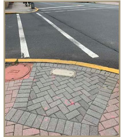
Figure 36. Curb ramps and standard crosswalks at the Evergreen Avenue intersection.
