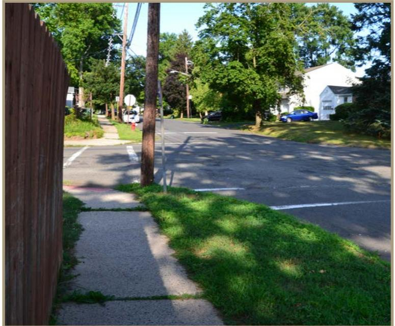
Figure 15. Missing curb cuts and ramps
