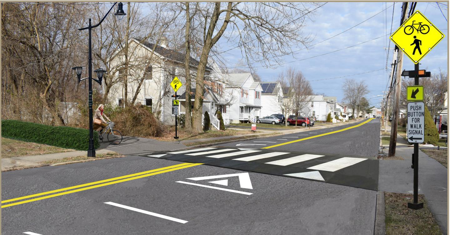
Figure 29. Photo simulation of proposed trail crossing on Lewis Street, looking east. Simulation shows a raised crosswalk, overhead lighting, and new pedestrian activated signage.
