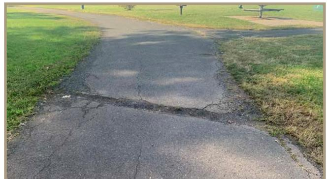
*Figure 49. Cracked walking trail.*
