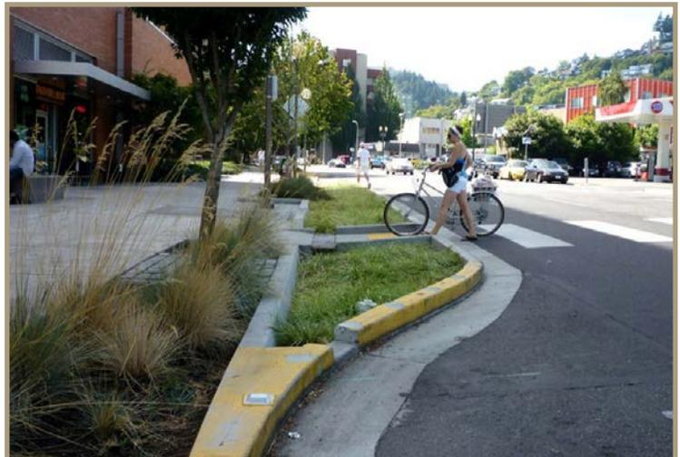
Figure 17. Green infrastructure used to narrow the roadway and provide a shorter crossing distance for pedestrians.
