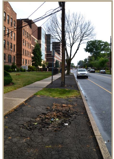
Figure 16. Unusable planting area due to unmaintained pavement.
