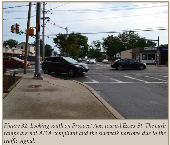
Figure 32. Looking south on Prospect Ave. toward Essex St. The curb ramps are not ADA compliant and the sidewalk narrows due to the traffic signal.
