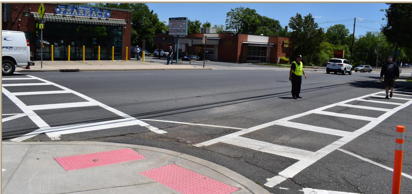
Figure 34. High visibility ladder crosswalks at Ford Avenue, looking eastward.
