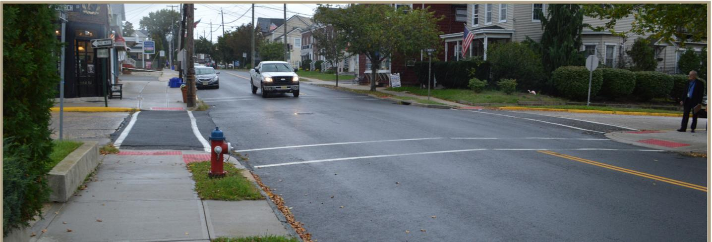
Figure 24. Fading crosswalks at the intersection of Main Street and Church Street, looking northwest on Main Street (photo taken before installation).
