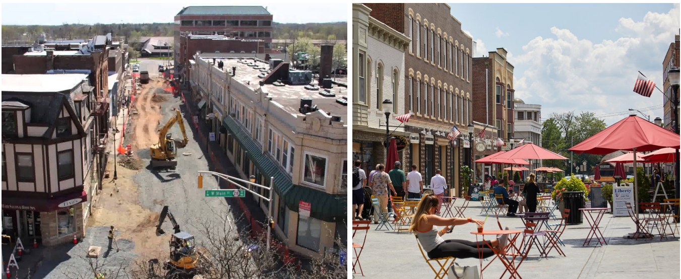
Figure 1. Reconstruction of Division Street in Somerville, NJ
