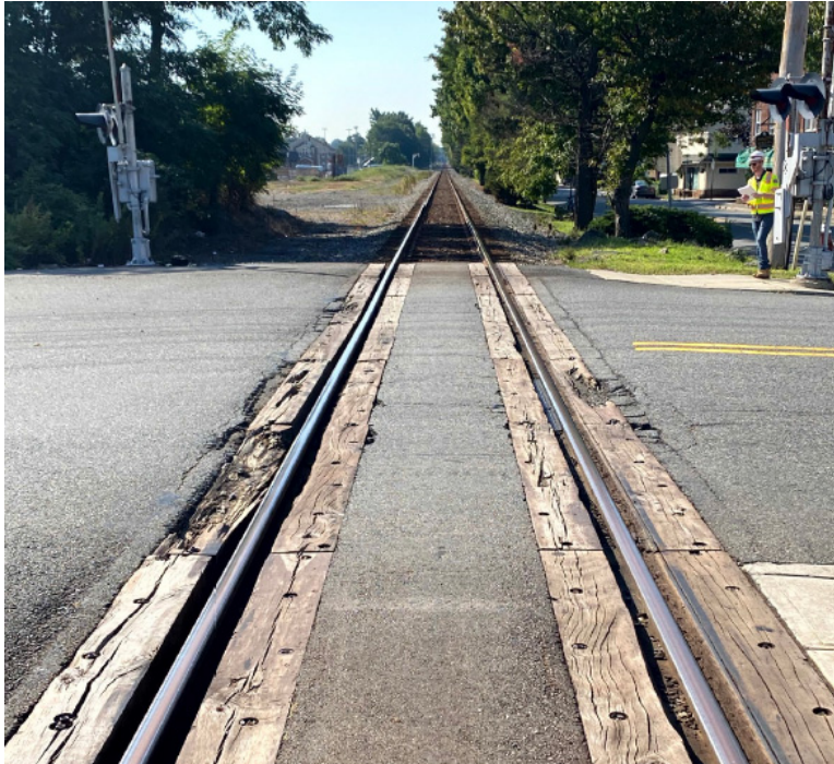
Figure 5.1 A Timber Flangeway Header in Poor Condition Can Be a Hazard to Cyclists
