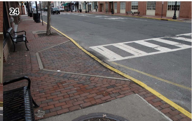
The northern half of Broad Street is finished with brick paver sidewalks that are generally in good condition. Brick paver curb ramps should be retrofitted with detectable warning surface. (RedBank_180201_093350.JPG, RedBank_180201_093439.JPG)
