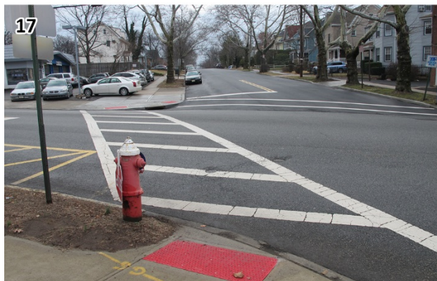
The skewed angles on the signalized intersection of Park Avenue and E. Pierrepont Avenue make it very difficult for pedestrians to read the traffic signals from the curb ramp. The signal may be considered for redesign or retrofitting with pedestrian signal heads and actuation.
