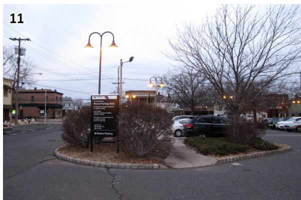
Lot 2 includes landscape islands with shrubbery in need of pruning. It may be possible to retrofit these islands to function as infiltration gardens by providing curb cuts and re-grading. (RedBank_180201_072330.JPG)
