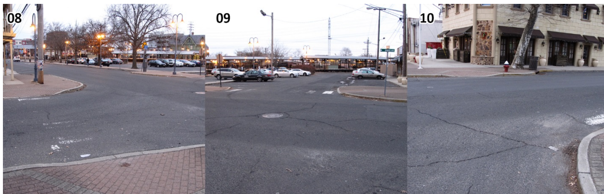
At the Bridge Avenue and Oakland Street intersection, all crosswalks need to be re-stripped. The northern leg of this intersection, crossing Bridge Avenue, did not include a crosswalk and curb ramps. It may be worth adding a crosswalk and curb ramps to this leg, since it is a natural travel pattern to/from the station. (RedBank_180201_071950.JPG, RedBank_180201_072000.JPG, RedBank_180201_072005.JPG)
