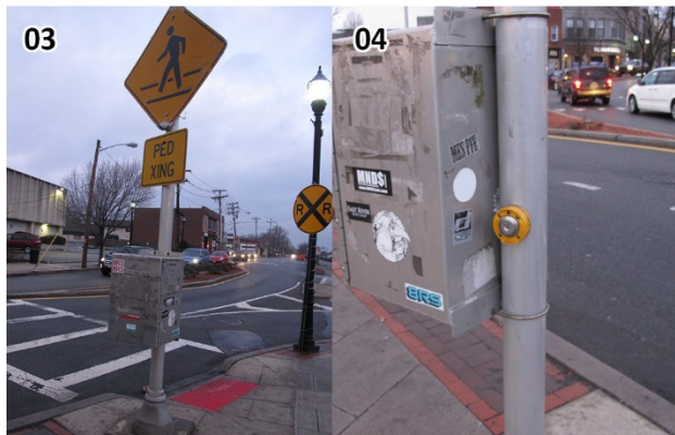
Pedestrian Crossing signs at the station along Erie Avenue include actuation devices but lack blinking signals. (Rutherford_180221_063646.JPG, Rutherford_180221_063720.JPG, Rutherford_180221_064215.JPG)
