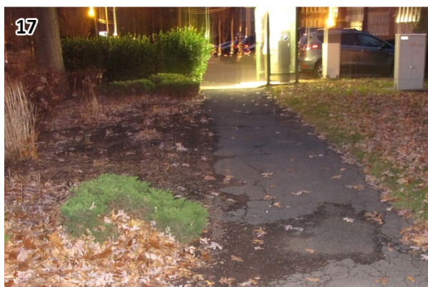
The asphalt path that provides access to Elm Street from Lot 9 is in poor condition. In the background, a large shrub is encroaching on the path near the pay station. (Summit_171206_165757.JPG)
