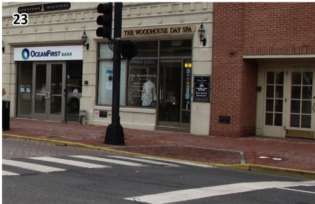
The northern half of Broad Street is finished with brick paver sidewalks that are generally in good condition. Brick paver curb ramps should be retrofitted with detectable warning surface. (RedBank_180201_093350.JPG, RedBank_180201_093439.JPG)
