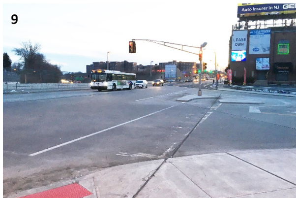
Crosswalk and other intersection markings do not adhere to the concrete roadway/bridge over the Garden State Parkway, leaving poorly marked intersections for all users.
