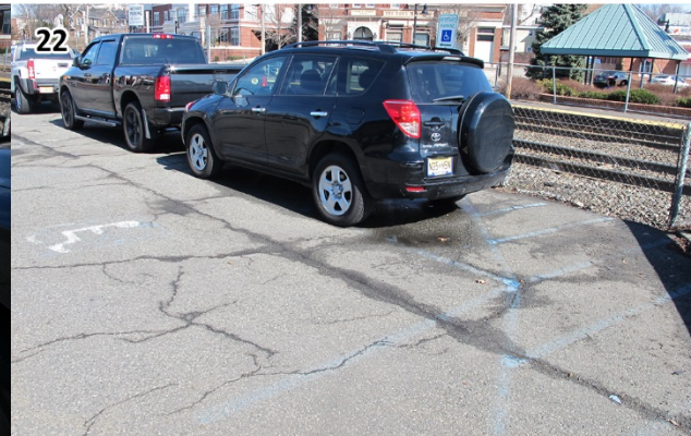
21 ADA parking in Lot 1 needs to be re-striped. The accessible way is provided only on the passenger side of the vehicle in this unique parallel parking situation. (Rutherford_180221_111319.JPG, Rutherford_180221_111332.JPG)
