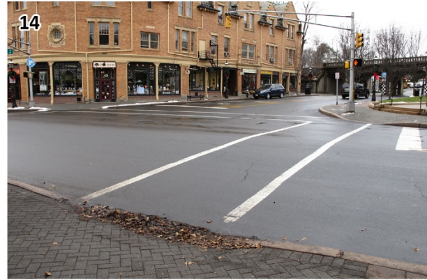
Crosswalks in the downtown business area generally lack tactile warning surface, as shown at Main Street and Green Village Road. (Madison_121217_114449.JPG)
