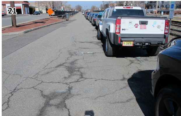
21 ADA parking in Lot 1 needs to be re-striped. The accessible way is provided only on the passenger side of the vehicle in this unique parallel parking situation. (Rutherford_180221_111319.JPG, Rutherford_180221_111332.JPG)
