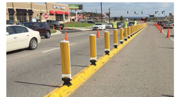
Example of modular lane separator curb with posts
