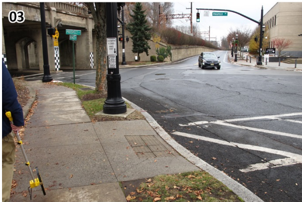
At Prospect Street and Kings Road, warning surfaces are concrete pavers set in a concrete field providing limited visual contrast. (Madison_121217_105614.JPG)
