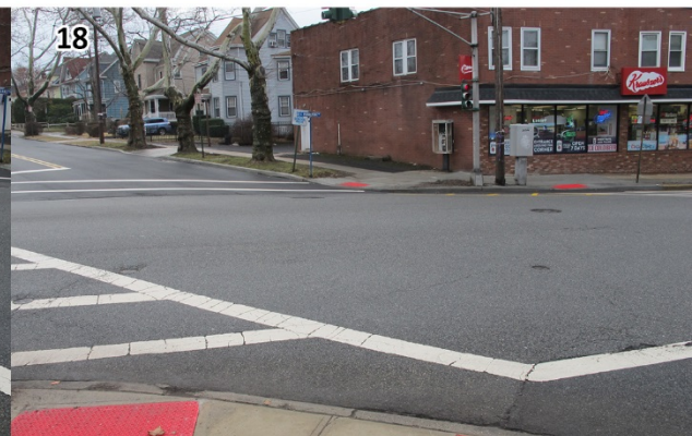
The skewed angles on the signalized intersection of Park Avenue and E. Pierrepont Avenue make it very difficult for pedestrians to read the traffic signals from the curb ramp. The signal may be considered for redesign or retrofitting with pedestrian signal heads and actuation.
