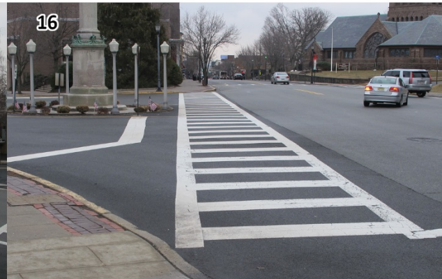
The unsignalized intersection of Park Avenue with Chestnut Street, W. Passaic Avenue, Lincoln Avenue, and E. Passaic Avenue is confusing for motor vehicles, bicyclists, and pedestrians. It features 7 crosswalk legs, the longest of which (shown) is about 160'. (Rutherford_180221_081117.JPG, Rutherford_180221_081212.JPG)
