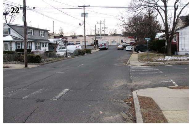
The intersection of Drummond Avenue and S. Bridge Avenue is an example of an intersection due for curb ramp replacement and crosswalk re-striping. (RedBank_180201_084825.JPG)
