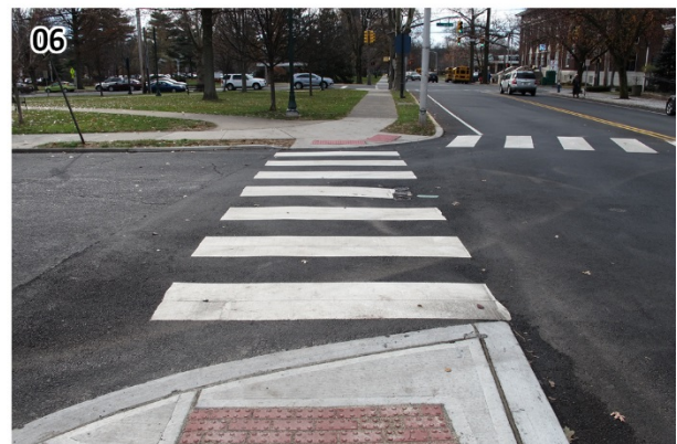
06 High visibility thermoplastic continental stripe crosswalks, as used at Maple Street and Railroad Avenue, offer the best combination of visual contrast and durability. (Summit_171206_104800.JPG)
