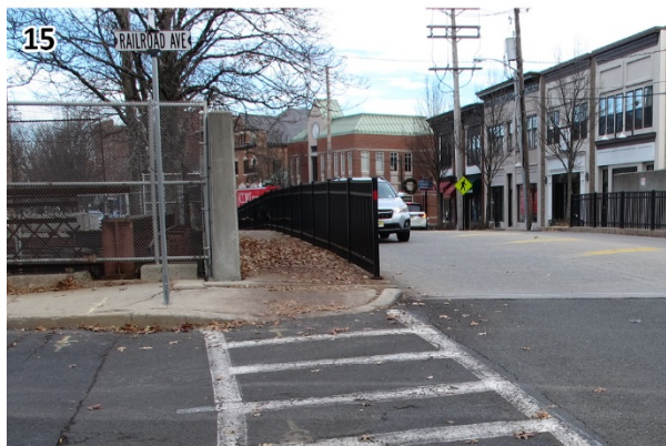
The curb ramp at Railroad Avenue and Summit Avenue is not ADA compliant. (Summit_171206_112621.JPG)
