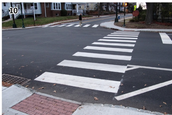
10 The curb ramps at Woodland Avenue & Springfield Avenue (and in most locations in Summit) are oriented to the tangent sides of the curb radius. (Summit_171206_161942.JPG)
