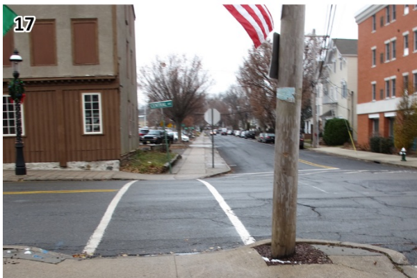
Tactile warning surface is absent from many curb ramps, such as observed at Central Avenue and Cook Avenue. (Newly reconstructed ramps were observed to include tactile warning surface). (Madison_121217_124134.JPG)
