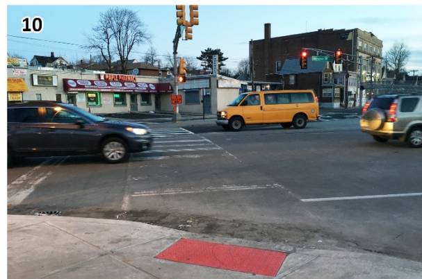
ADA compliant ramps are found on most intersections adjacent to the bus terminal, but crosswalk markings are often faded due to high traffic volumes.
