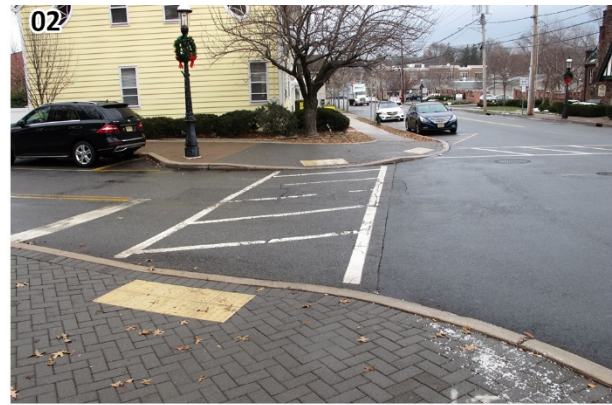
At Prospect Street and Lincoln Place, yellow warning surfaces against the gray paver field provide some visual contrast. (Madison_121217_110119.JPG)
