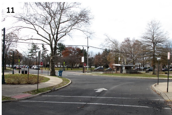
11 The southeast crossing of Railroad Avenue to Summit Station would benefit from upgrades to the crosswalk and curb ramp. (Summit_171206_110857.JPG)
