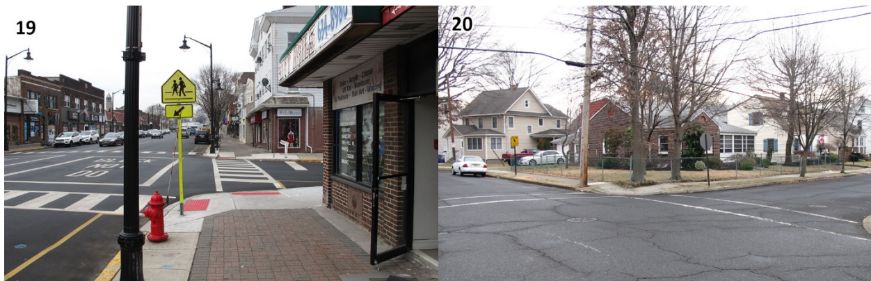
Crosswalks and curb ramps varied in condition throughout the study area. It is generally recommended to bring all curb ramps up to standard in terms of slope and inclusion of detectable warning surface. (Woodbridge_180122_095742.JPG, Woodbridge_180122_093500.JPG)
