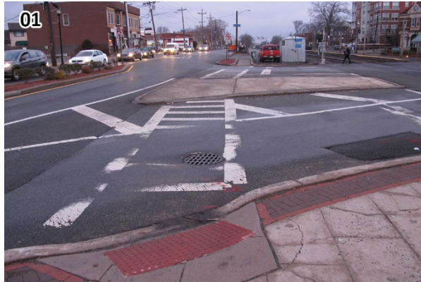
Crosswalks connecting Lot 1 (background) with the station are in poor condition. (Rutherford_180221_063443.JPG)
