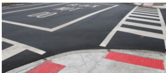
High visibility crosswalks with ADA-compliant curb ramps and detectable warning strips
