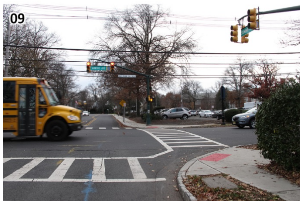
09 The curb ramps at Summit Avenue & Morris Avenue are oriented to the apex of the curb radius. (Summit_171206_151648.JPG)
