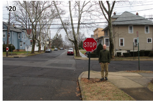
20 Most of the stop signs in residential areas were observed to have a mounting height of 5'. Mounting height should increase to 7' minimum. Add appropriate plaques to indicate two-way or all-way stops. (Rutherford_180221_091323.JPG)
