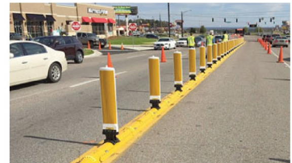
Example of Flexible Delineators (above) and modular lane separator curb with posts (below)
