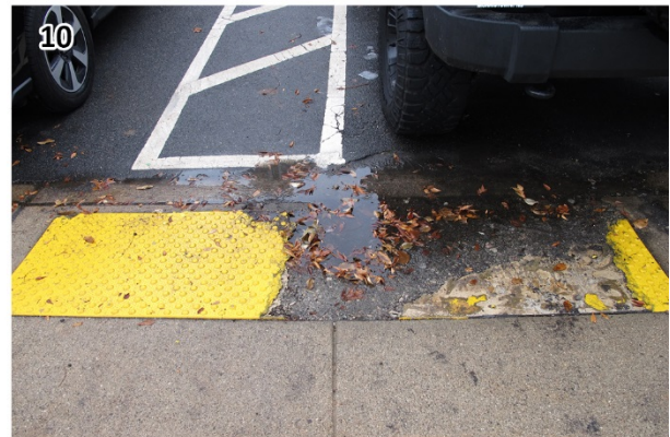
The pedestrian ramp into Lot 1 at the Kings Road and Maple Avenue entrance is in disrepair. (Madison_121217_104538.JPG)
