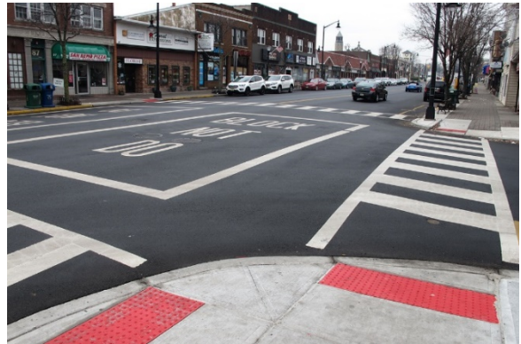
Curb ramps leading to ladder style crosswalks near Woodbridge Station
