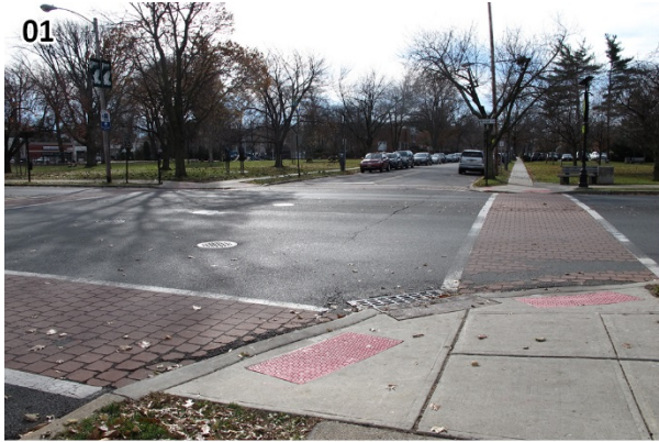
01 Stamped asphalt crosswalks at Elm Street and Broad Street are showing wear. (Summit_171206_105720.JPG)
