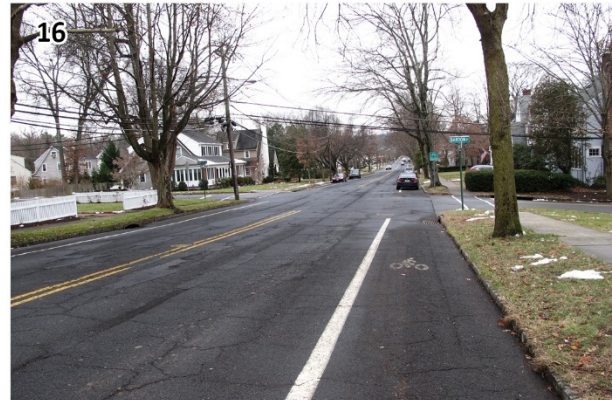
The view south on Greenwood Avenue at Bardonia Street shows an example of the striped shoulder with bicycle blaze that is used around the borough. (Madison_121217_122151.JPG)
