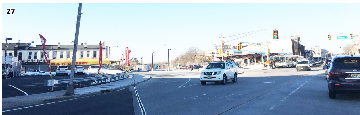
The intersection of Washington Avenue, Springfield Avenue and Cleremont Street also sits on a bridge over the Garden State Parkway. Standard paint markings over the concrete roadway wears quickly and has left the intersection difficult to navigate.
