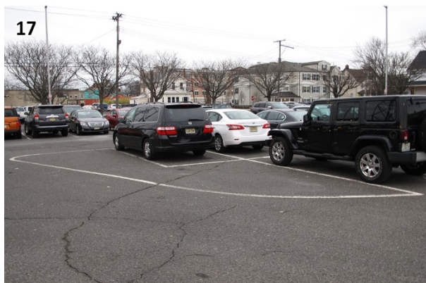
Lot 3 includes striped parking lot islands. These can be retrofitted as infiltration gardens through pavement removal, curbing, soil amendment, and planting. (RedBank_180201_074922.JPG)
