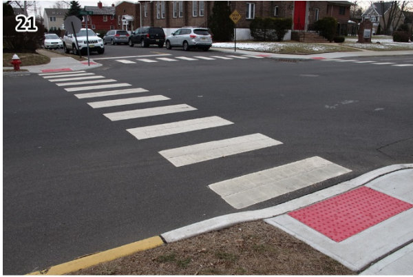
The Bridge Avenue and Herbert Street intersection is an example of ADA-compliant curb ramps and high visibility crosswalks that could be replicated throughout the borough. (RedBank_180201_084125.JPG)
