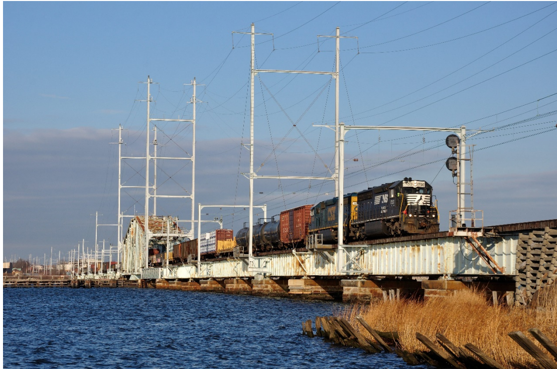
Figure 6-8. Conrail Freight Train on Amboy Corridor near Perth Amboy
