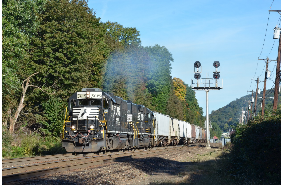
Figure 6-3. NS Freight Train on HX Corridor near Suffern, NY
