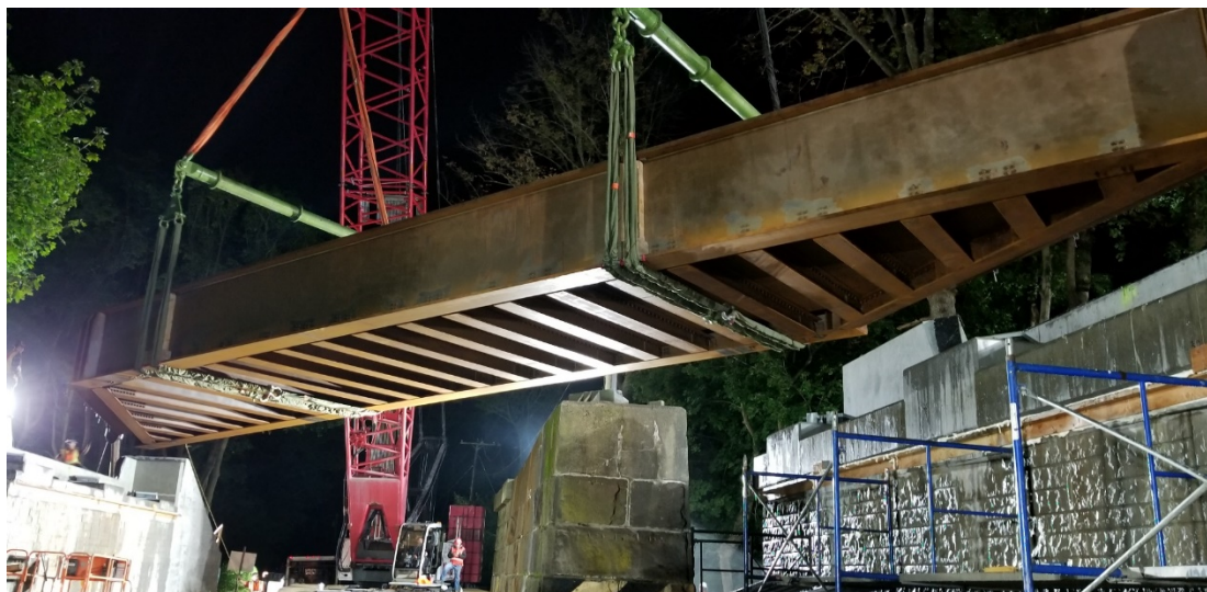
Figure ES-5. Example of a Superstructure Replacement
