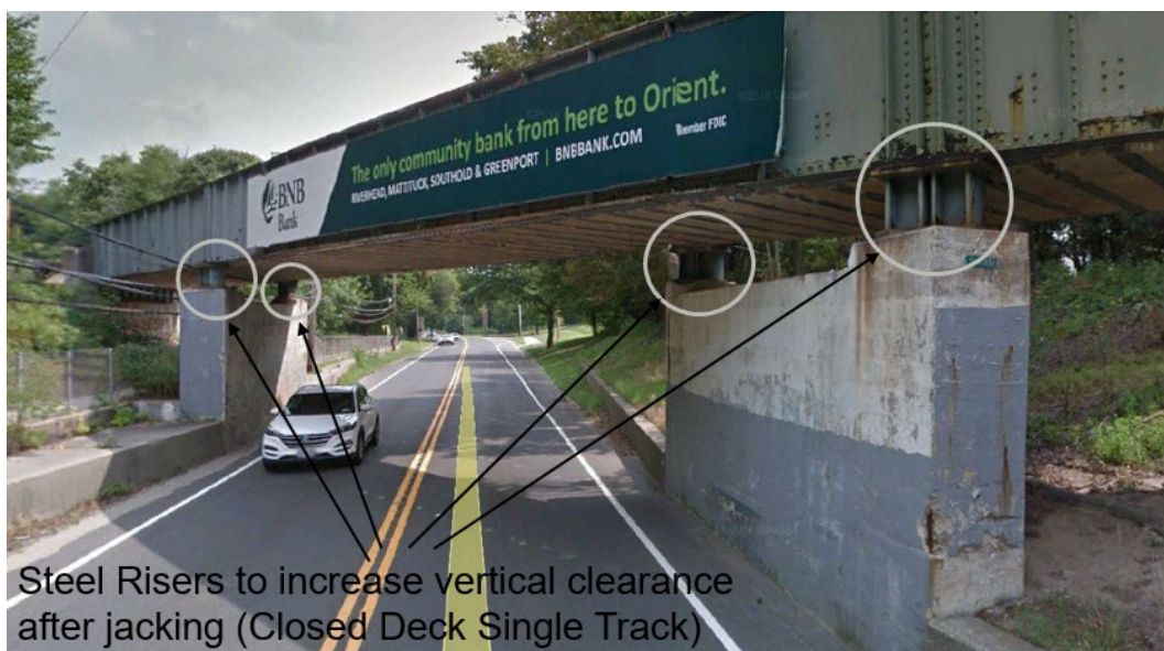
Figure ES-6. Raised Superstructure
