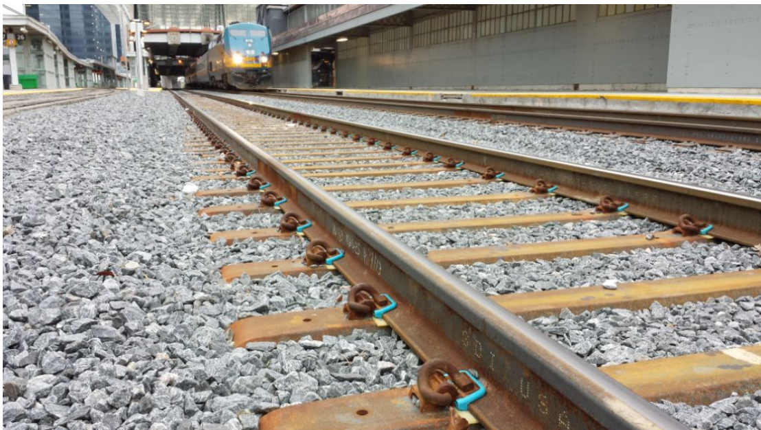
Figure 2-5. Example of Implementation of Steel Ties and Undercutting
