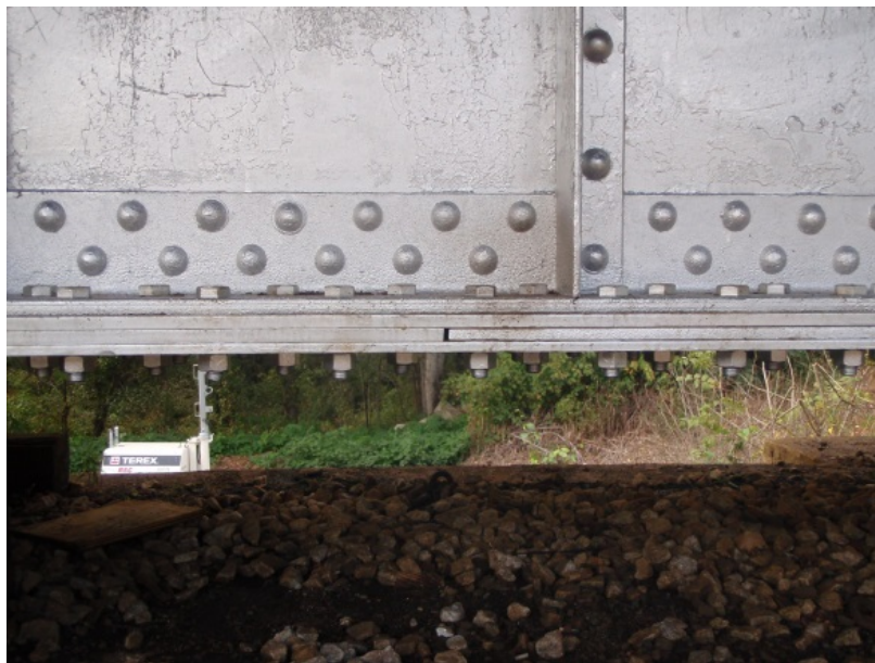
Figure 5-4. Example of Built-up Steel Girder Section Showing Flange Cover Plates
