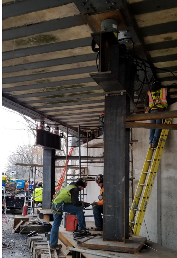
Figure 2-4. Superstructure Being Jacked with Hydraulic Jacks
