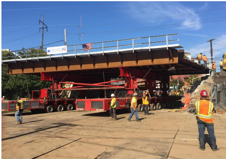
Figure 5-5. Triple Track Superstructure Replacement using SPMT in Weekend Rail Outage
