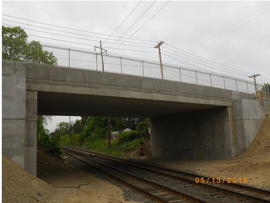
Figure 5-3, Overhead Bridge Replacement with Increased Vertical Clearance on Long Island Rail Road Mainline
