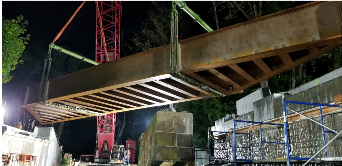
Figure 2-1. Example of a Superstructure Replacement
