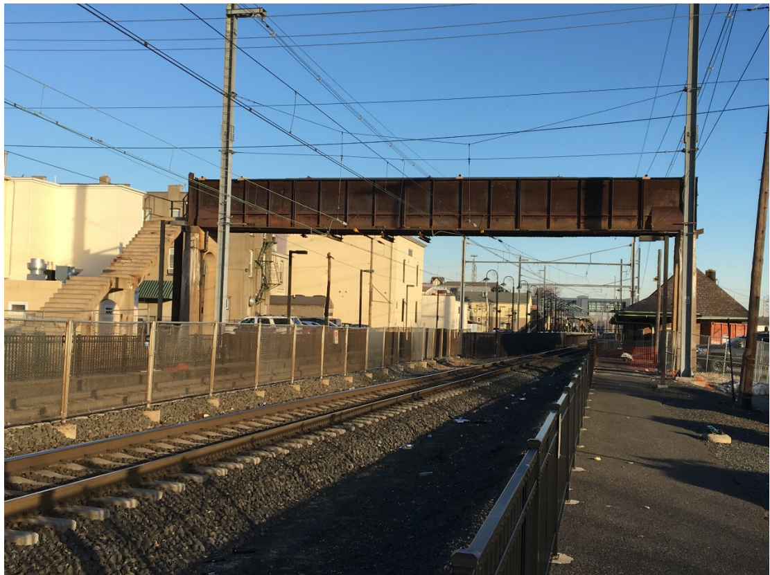
Figure ES-4. Geometric Restriction Pedestrian Overpass on Coast Line Corridor
