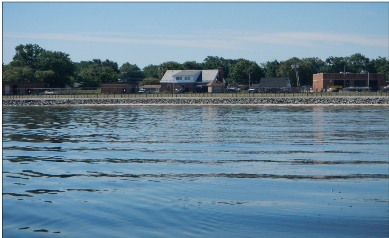
Photo 2 – Property at east end of site is protected by a concrete seawall and rip rap revetment.
