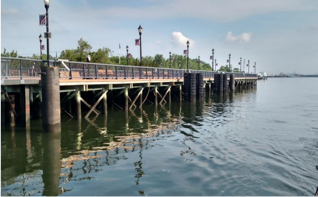
Carteret Waterfront – New Timber Pier with Breasting Panels and Hardware for Mid-Sized Vessel Berthing Capabilities
