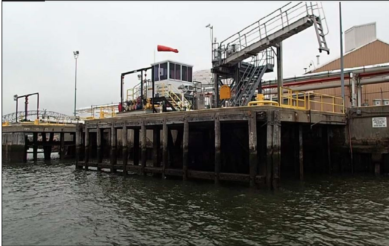
Photo No. 1 – Main loading platform supported by steel pipe piles.
