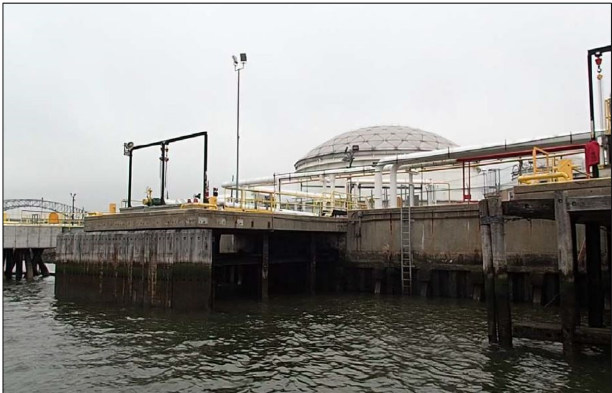
Photo No. 2 – Secondary pipe pile supported loading platform.
