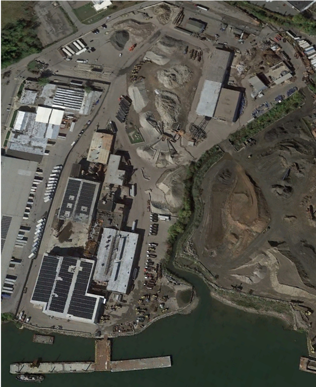
Bayshore Recycling Center Site Detail with "T" Pier – Image from Google Earth
