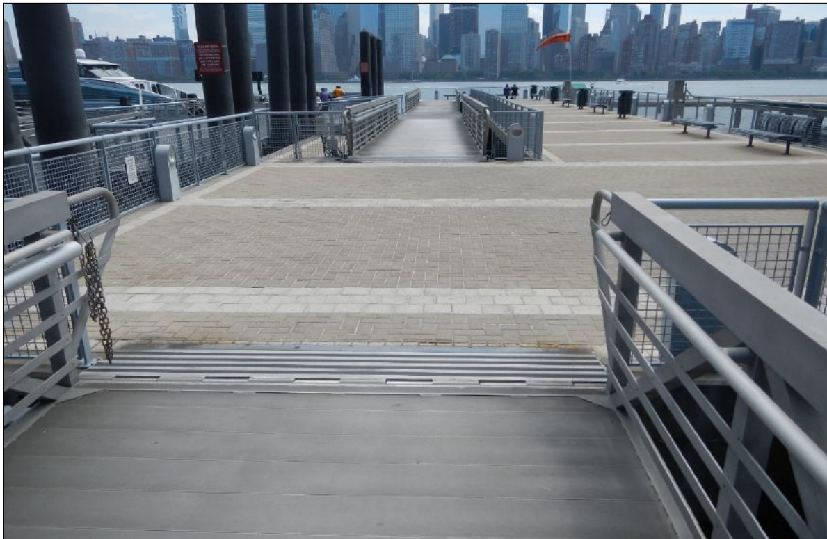
Photo No. 2 – Pedestrian access.
