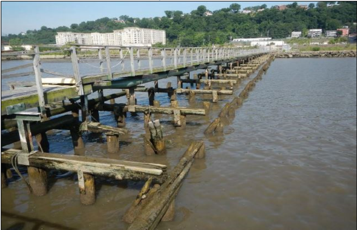
Hess Tank Farm – Timber Access Trestle and Pipe Rack
