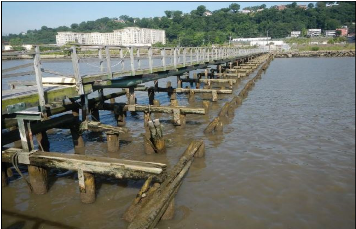
Photo No. 2 – Timber access trestle and pipe rack.
