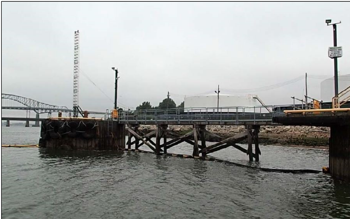
Photo No. 2 – South Breasting Cell and timber supported access trestle.
