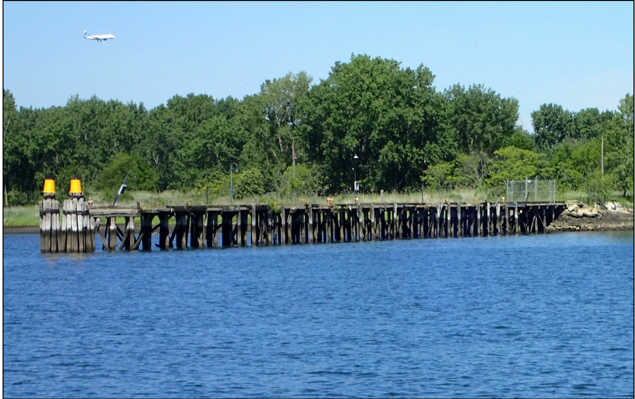
Photo 1 – Timber pier at north end of site.
