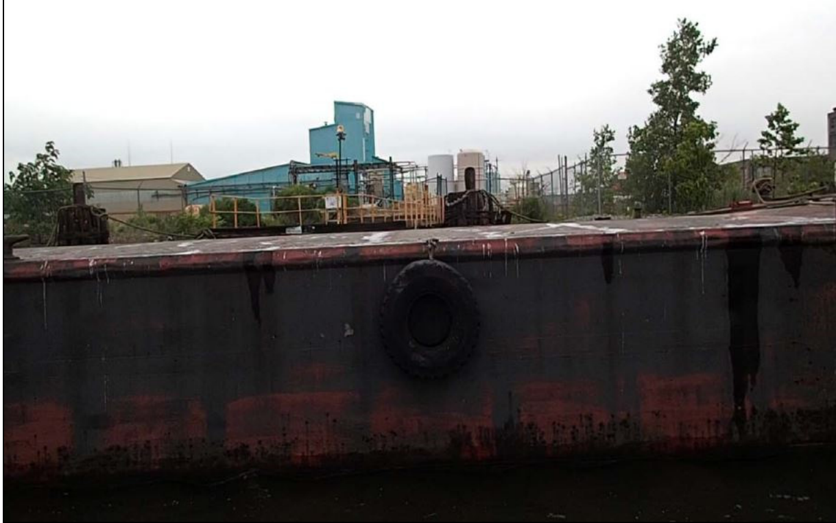
Photo No. 1 – Main breasting platform and trestle. Barge moored at berth.
