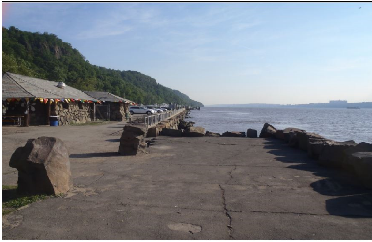
Photo No. 2 – View to north from abandoned landing. Commercial business located inshore of seawall.
