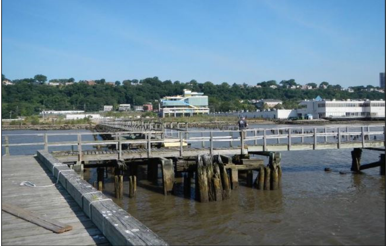
Photo No. 1 – Main timber berthing and transfer platform.
