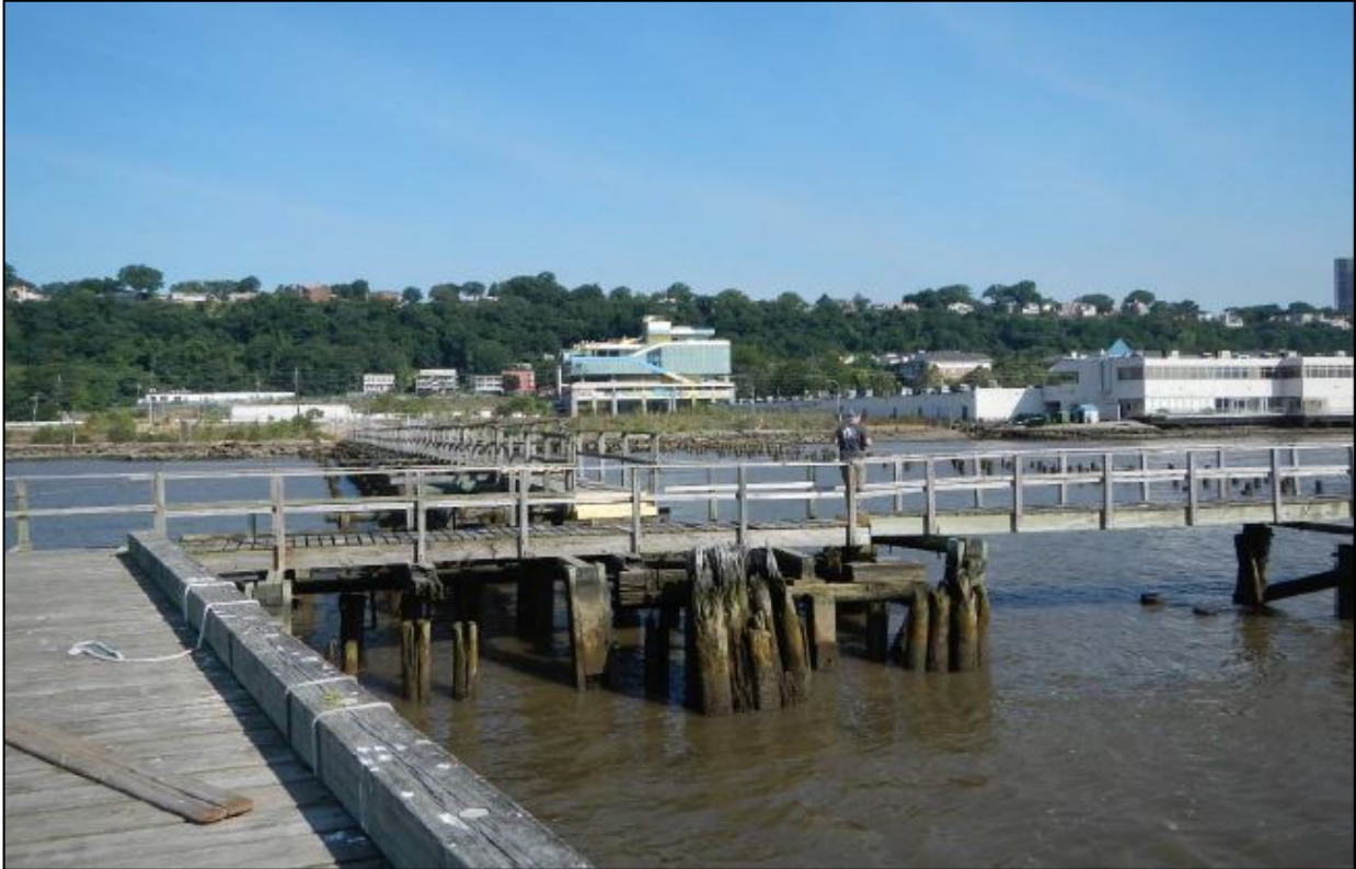
Hess Tank Farm – Main Timber Berthing and Transfer Platform
