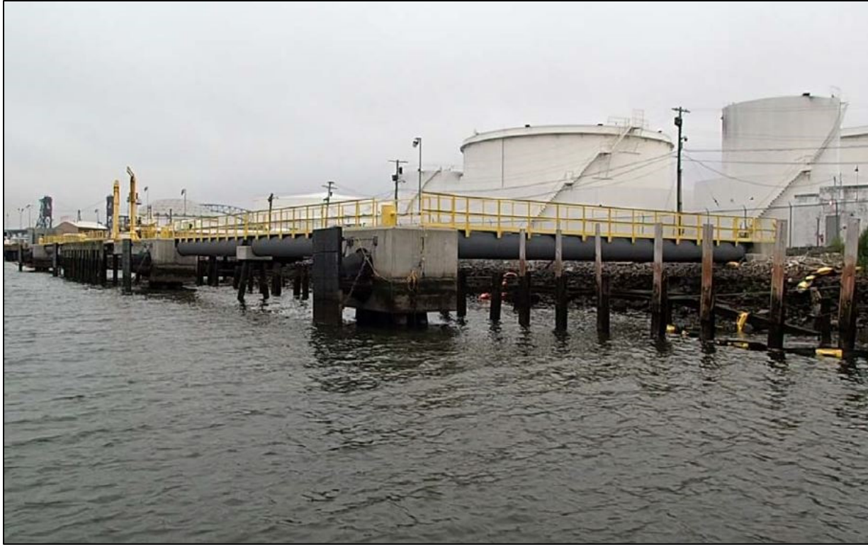
Photo No. 1 – Pipe supported trestle connecting platforms.
