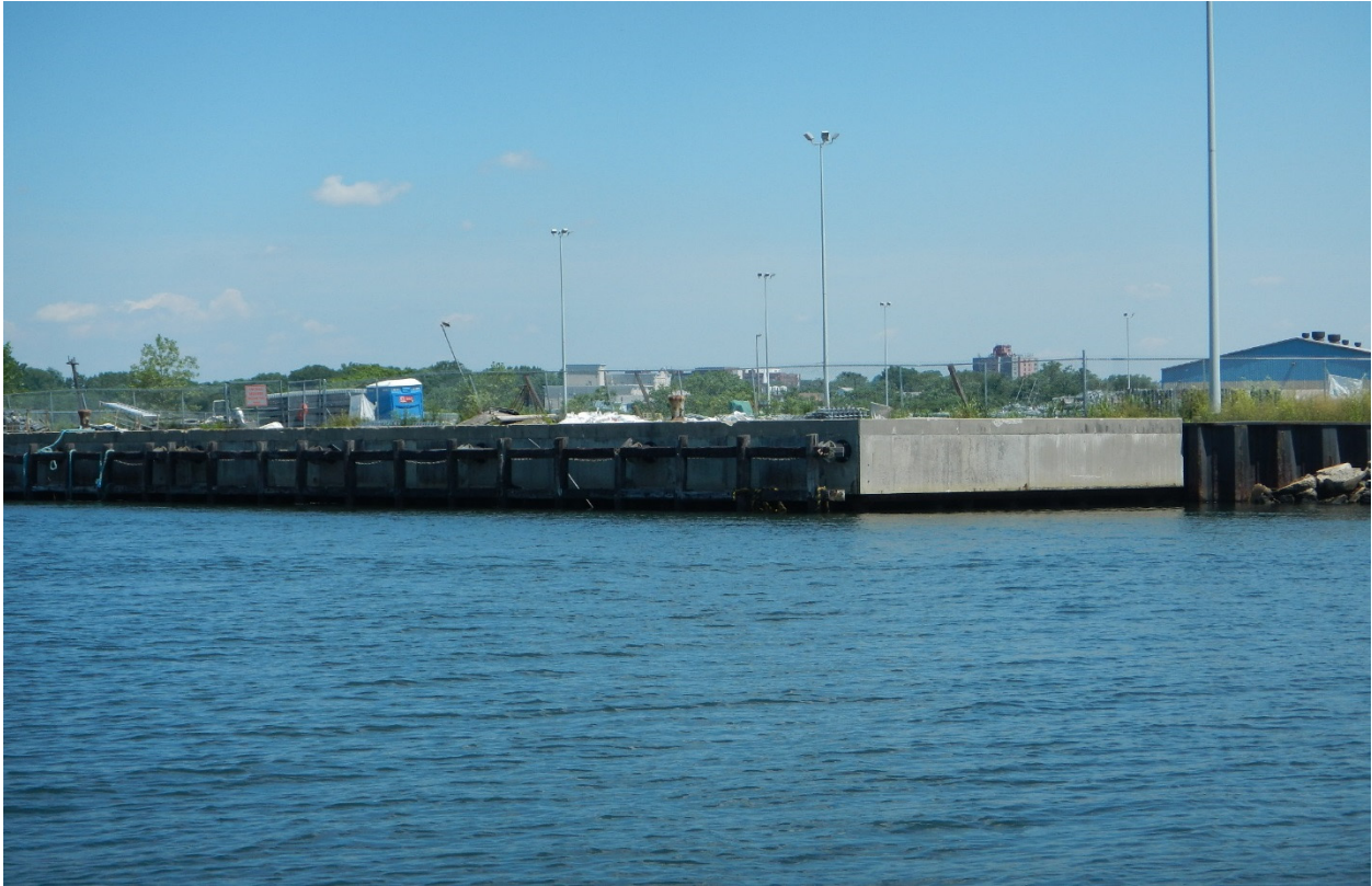
Photo 1 – Pipe pile supported concrete wharf with timber fender system intact
