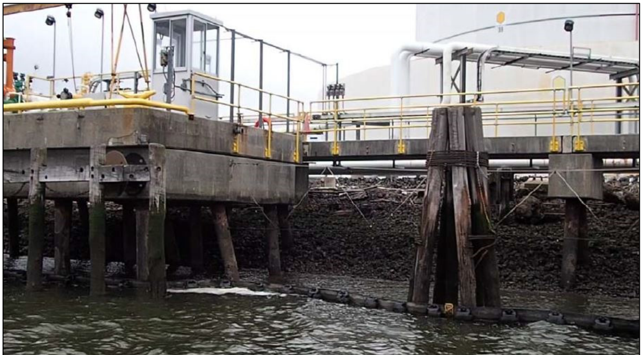
Photo No. 2 – North breasting platform.
