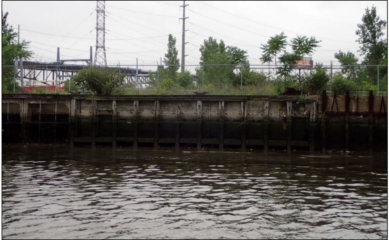
Photo No. 1 – Concrete bulkhead at the south end of the site.
