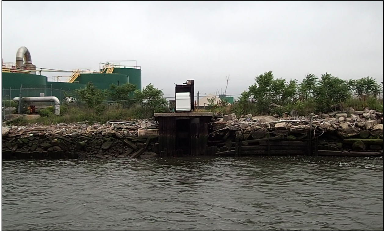
Photo No. 1 – Abandoned intake structure at north end of berth.
